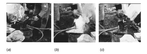
**Figure 7.20** Exothermic bonding is the preferred method of joining the elements of a ground system. This photo sequence illustrates the procedure: (*a*) the powdered copper oxide and aluminum compound are added to the mold after the conductors have been mechanically joined; (*b*) final preparation of the bond before igniting; (*c*) the chemical reaction that bonds the materials together.
