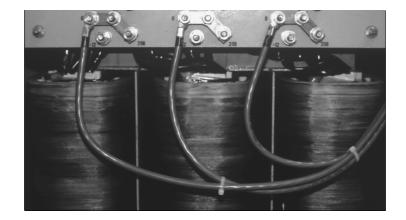
Figure 4.29 A medium-power, 3-phase transformer.
