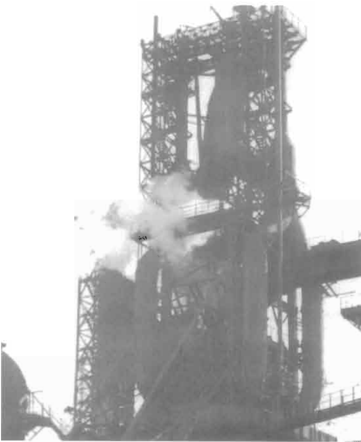
Figure 10. Shows air emissions from blast furnace operations.
