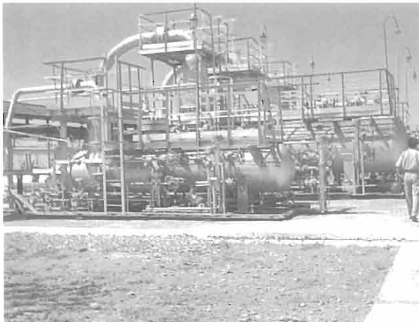
Figure 16. Gas processing plant.
