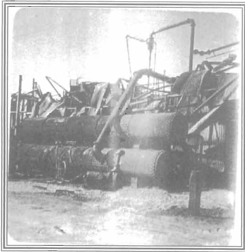
Figure 15. Destroyed penta vessels from fire.
