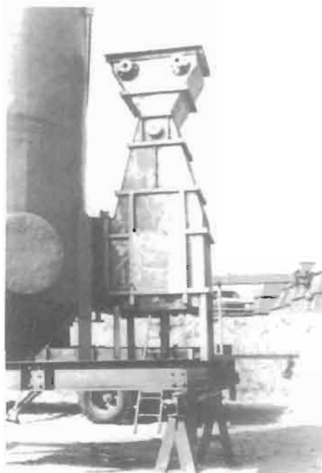
Figure 19. Variable venturi scrubber for flyash and sulfur dioxide removal.
