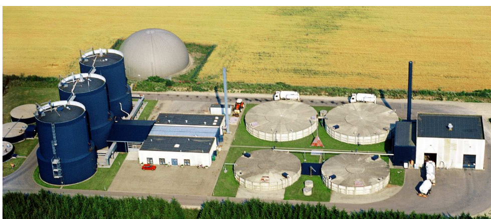
Figure 4.8 Picture of centralised co-digestion plant in Denmark (LEMVIG BIOGAS)
