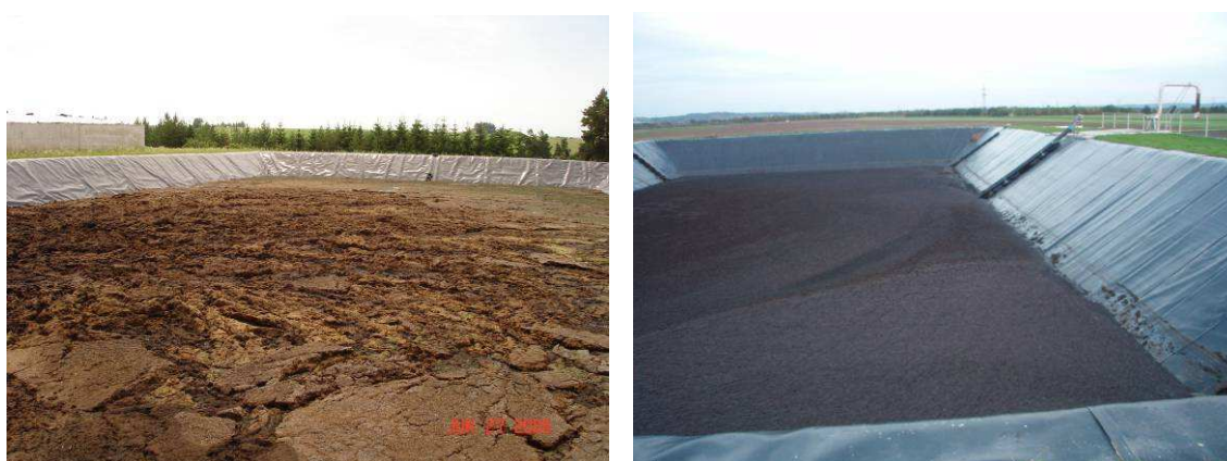
Figure 7.34 Open pond lagoons for digestate storage (AGRINZ 2006)
