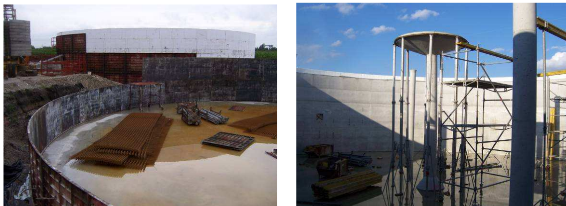
Figure 7.19 On-site construction of vertical digesters (RUTZ 2007)
