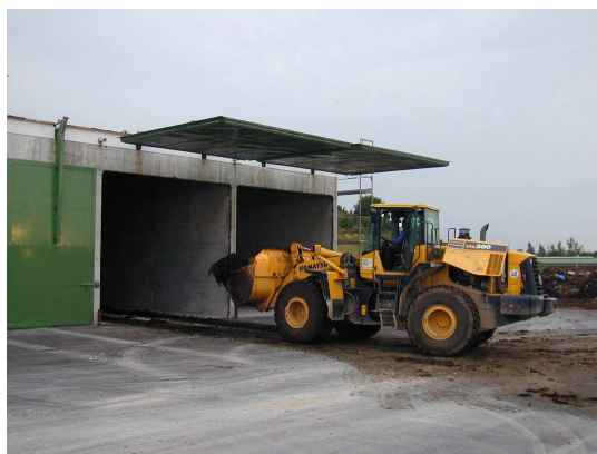
Figure 7.18 Garage-type batch digester, loaded by a loader (BEKON 2004)
