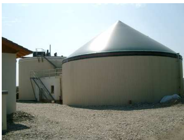
Figure 4.7 Vertical digester in Germany, built in 2005 for digestion of energy crops (KRIEG and FISHER 2008)
