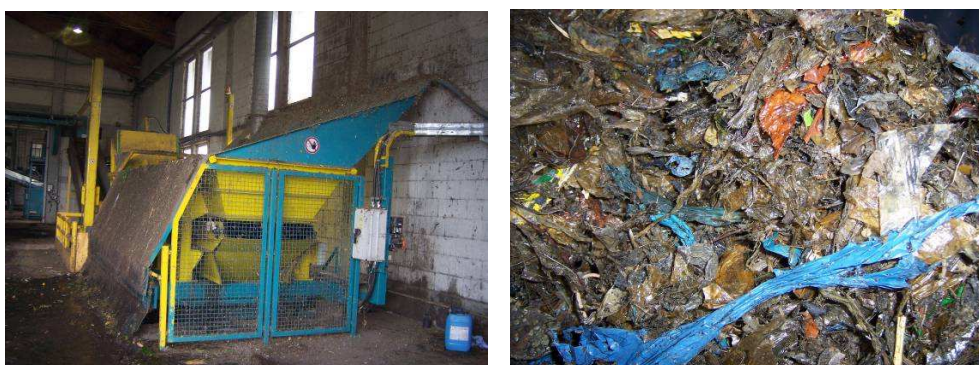
Figure 7.7 Feed-in system for cleaning municipal solid waste ( left ) and “problematic material” which was separated from catering wastes ( right ) (RUTZ 2007)
