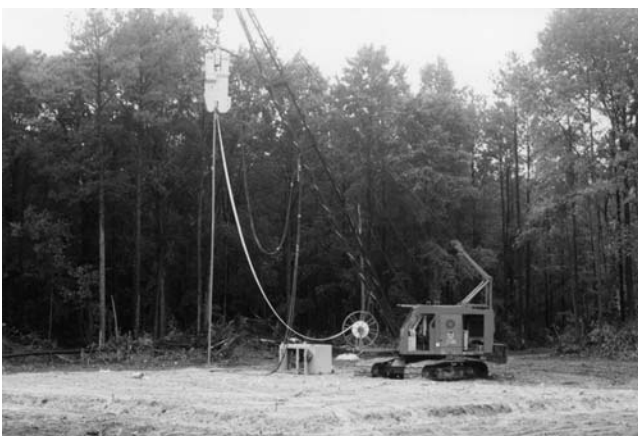
FIGURE 39.35 Wick-drain installation.
