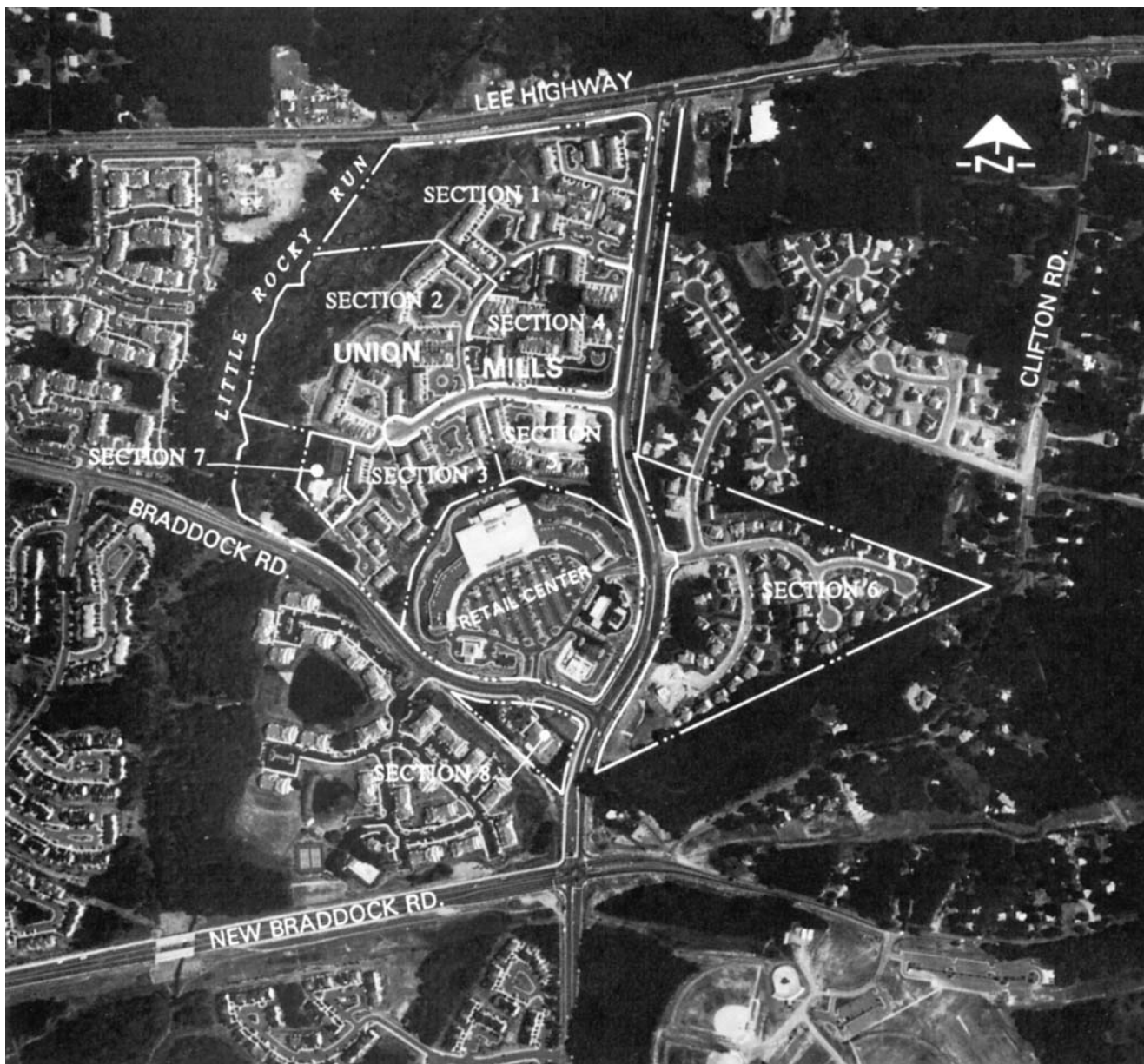
FIGURE 40.22 Union Mills site (circa 1993). Courtesy of Air Survey Corporation, Sterling, Va.
