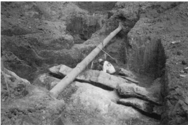
FIGURE 39.32 (a) Surface collapse (b) Preparing bedrock for remedial measures.
