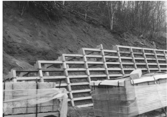
FIGURE 39.23 Photo of a cribblock wall.
