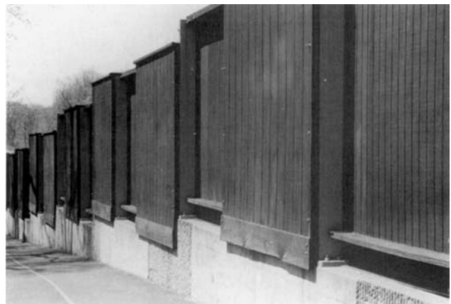
FIGURE 19.8 Noise barrier: wood.
