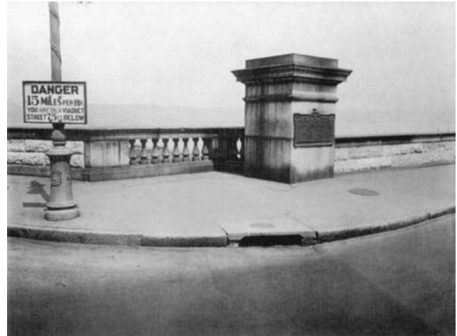
FIGURE 18.5 Riverside Drive Viaduct (124th Street southwest, circa 1927).
