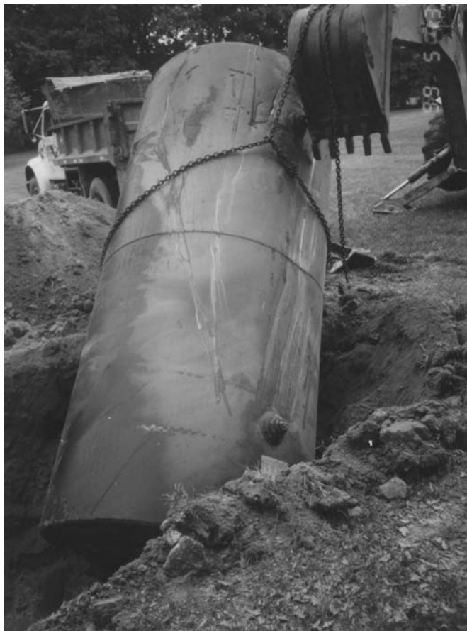
FIGURE 8.3 Removal of leaking underground storage tank.
