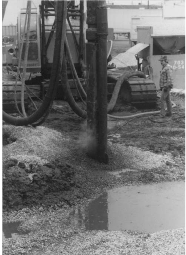
FIGURE 39.33 Vibro-replacement ground-improvement method using stone columns.
