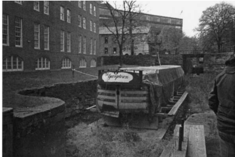
FIGURE 18.2 Photo of C&O Canal lock reconstruction.
