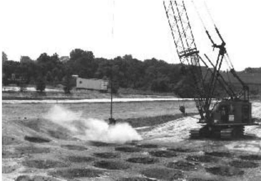
FIGURE 39.34 Dynamic compaction. (Courtesy of Terasystems, Inc.)
