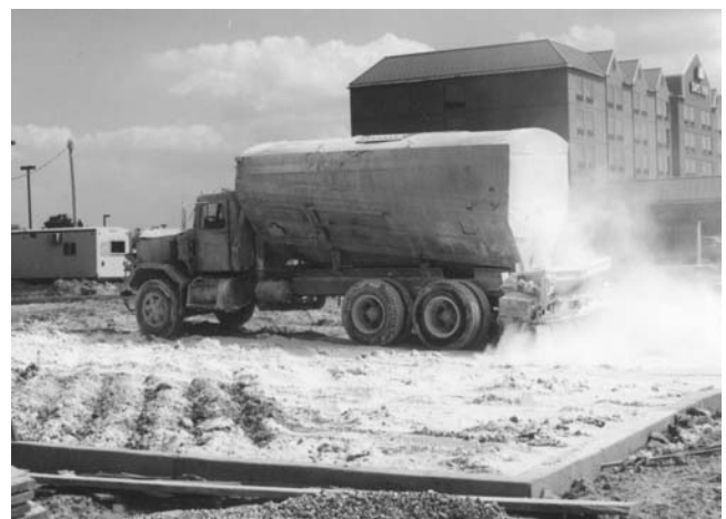
FIGURE 39.36 Lime stabilization of clayey subgrade soils in a proposed parking lot.
