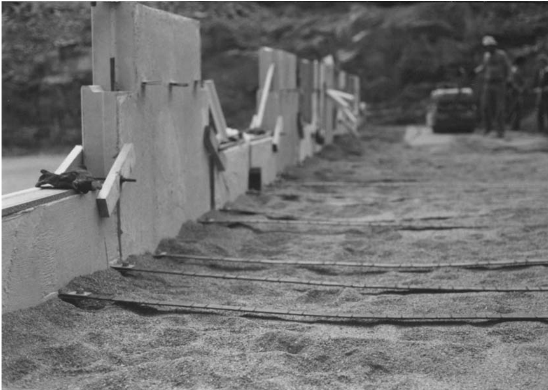
FIGURE 39.21 Photo of reinforced earth wall showing pre-fabricated concrete facing panels, galvanized metal reinforcing strips, and granular backfill.
