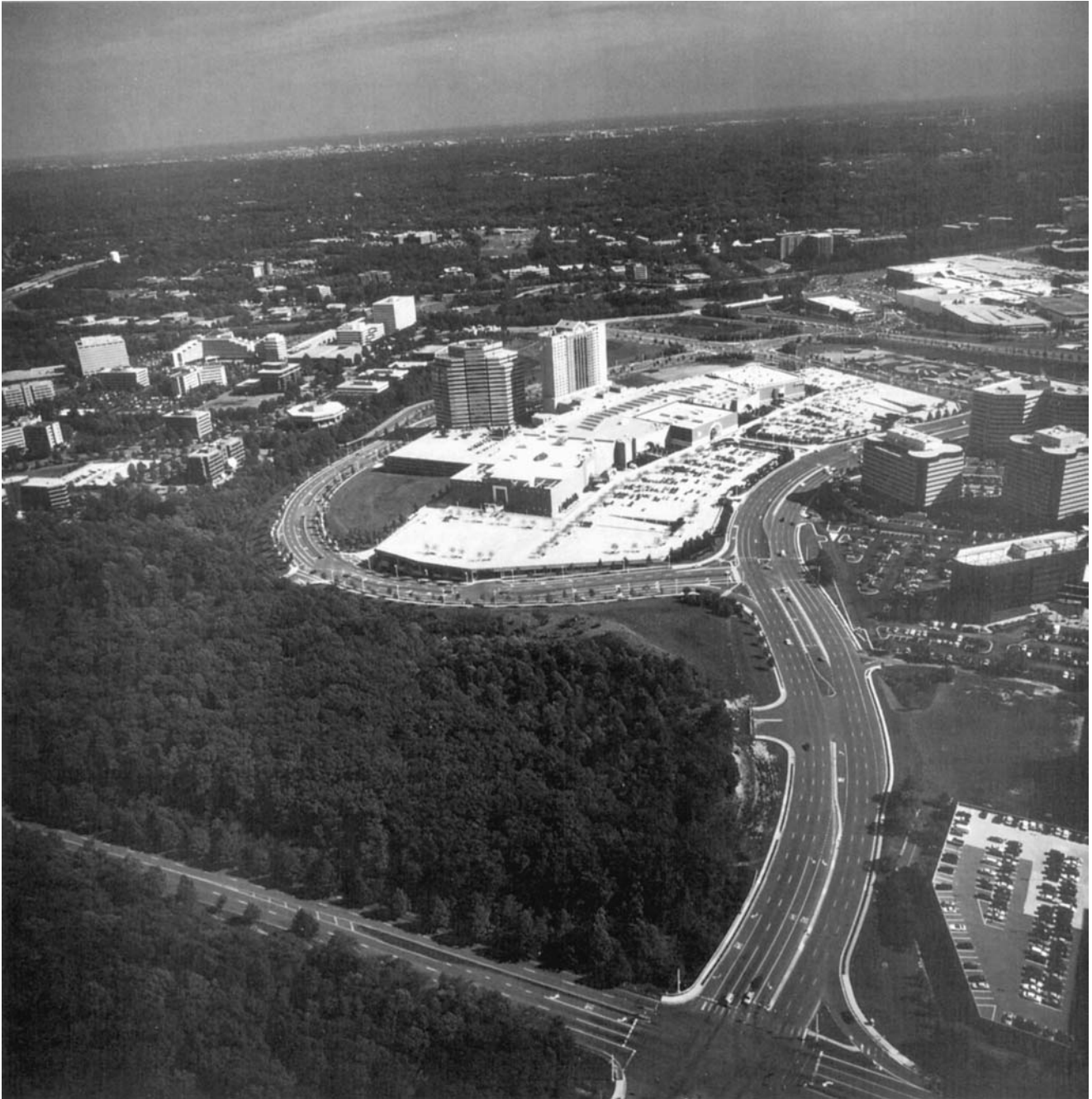
FIGURE 12.23 Retail mall with structured parking. (Photo by Larry Olsen)
