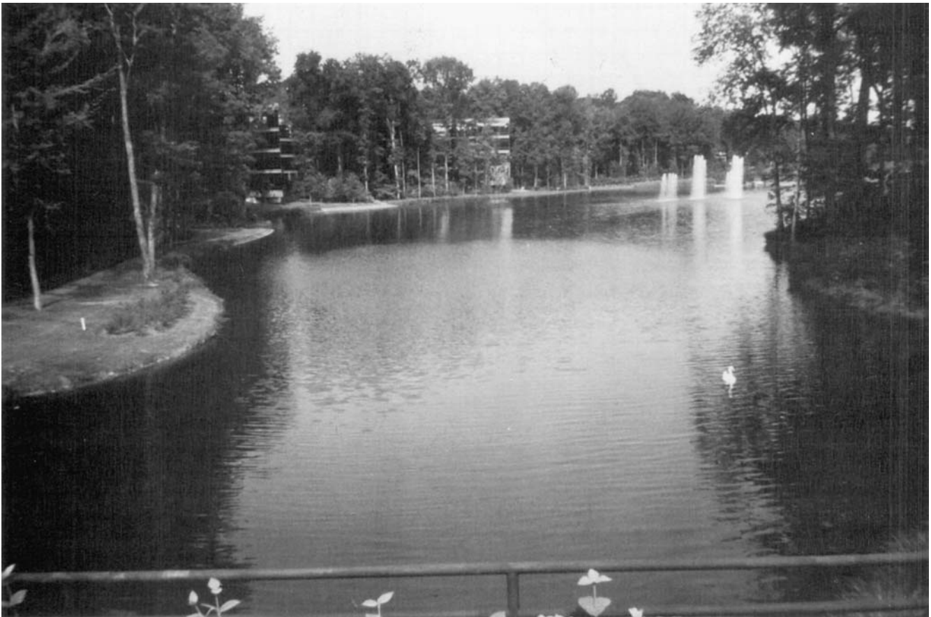
FIGURE 22.13 The use of a stormwater management facility as an amenity is exhibited in this permanent pond at Fair Lakes, a major mixed-use project in Fairfax Co. Extensive trees and area supplemented with additional landscape materials provide a varied edge environment and reinforce the water jet features with an attractive setting for the proximate office buildings. The facility likewise provides a rich visual experience as viewed from the pedestrian path (left) and adjacent roadway (upper right). The spillway riser structure behind the water jet is shown in Figure 22.16.
