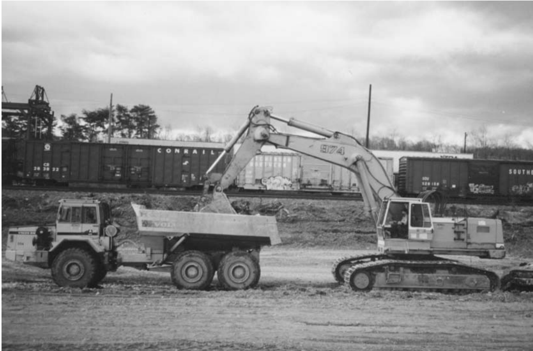
FIGURE 24.1 Grading the site. (Photo Courtesy of Christer Carshult)
