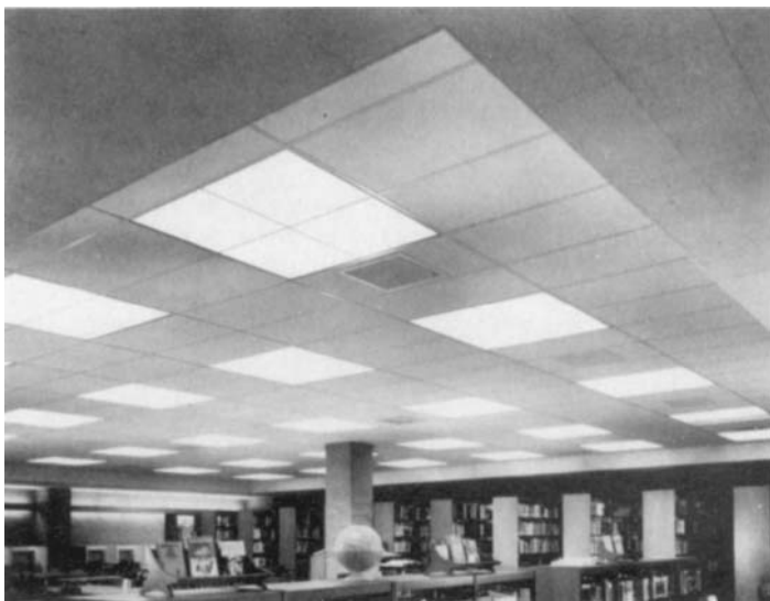
FIGURE 11.98 Library ceiling comprising both acoustical panels and acoustical tiles, integrated with lighting panels. ( U.S. Gypsum Company. )
