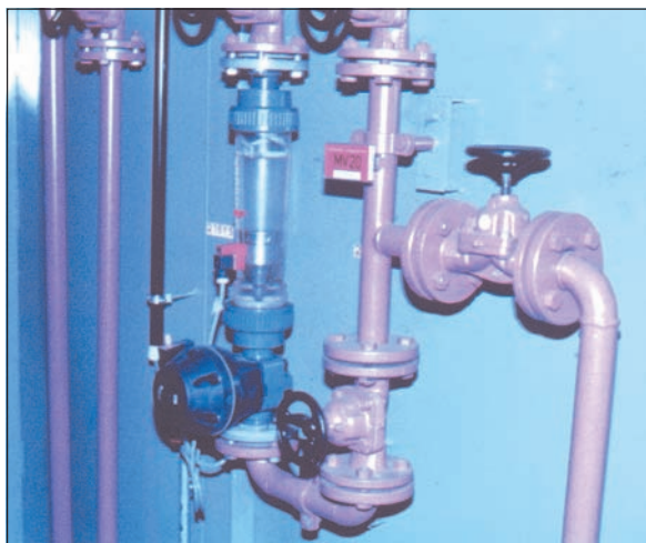
Fig. 4.2.89 Picture and scheme of volume flow meter by floats
