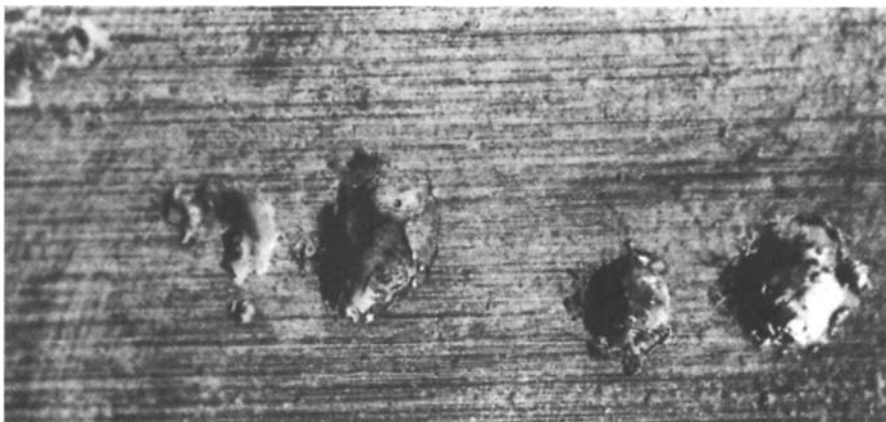
Figure 2.86 The craters on working surface caused by electric current flow.
