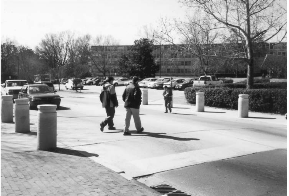
FIGURE 14.4 A speed table can help slow vehicles, providing for a safer pedestrian crossing. (Source: Daniel L. Carter.)
