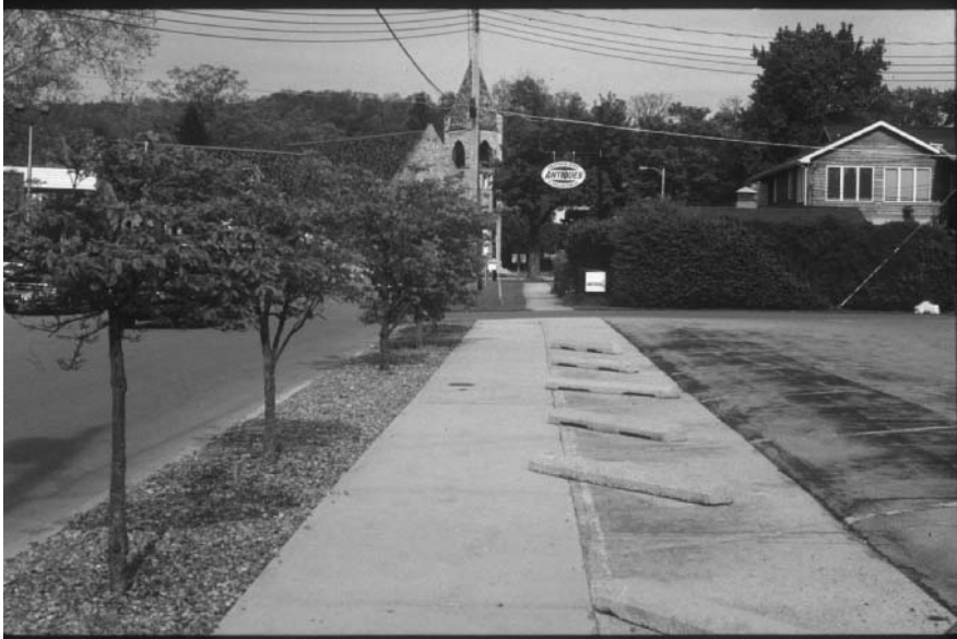
FIGURE 21.3 Wheelstops from parking lot intruding onto and near sidewalk, creating tripping hazard for pedestrians.
