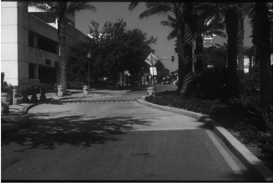
FIGURE 21.8 Mid-block crossing connecting parking structure with downtown retail mall.
