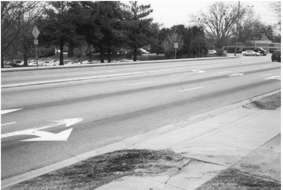
FIGURE 14.3 A narrow, raised median helps treat a safety problem created by a driveway near a major intersection. (Source: Daniel L. Carter.)
