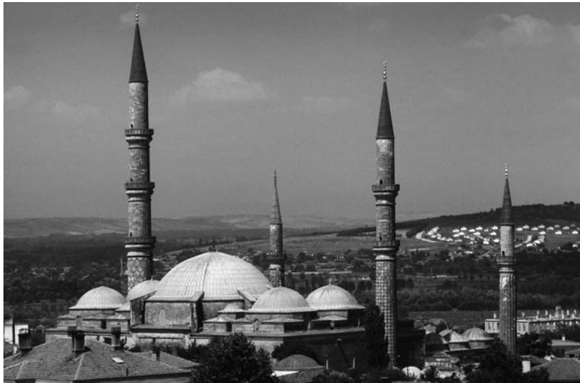
Figure 8.9 (a, b) Üç Şerefeli Cami, Edirne, plan (after Kuran, Mosque , p. 177, courtesy University of Chicago Press) and view of covering showing arrangement of prayer hall domes (Photo Walter B. Denny)
