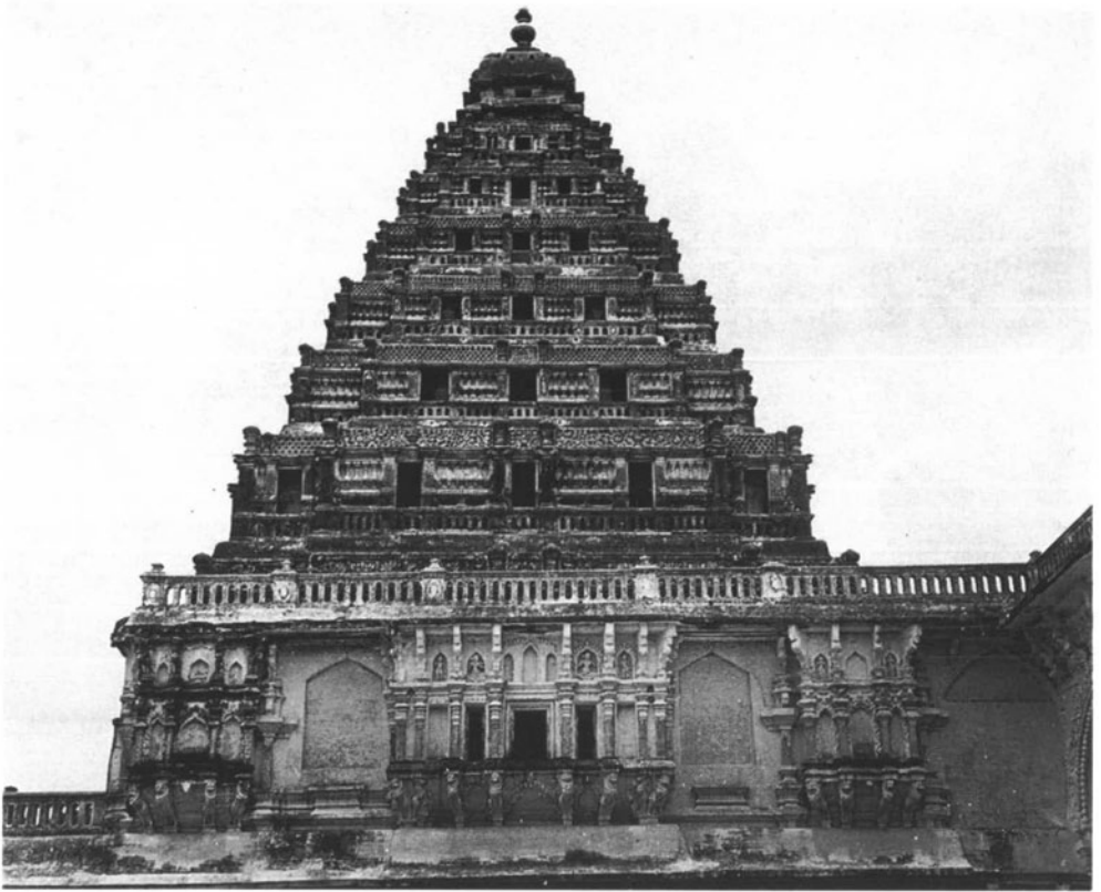
107 Tower, Thanjavur, seventeenth century
