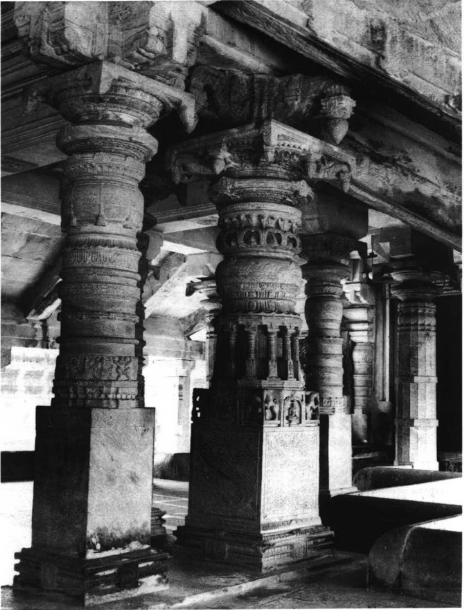
31 Mandapa columns, Chandranatha Basti
