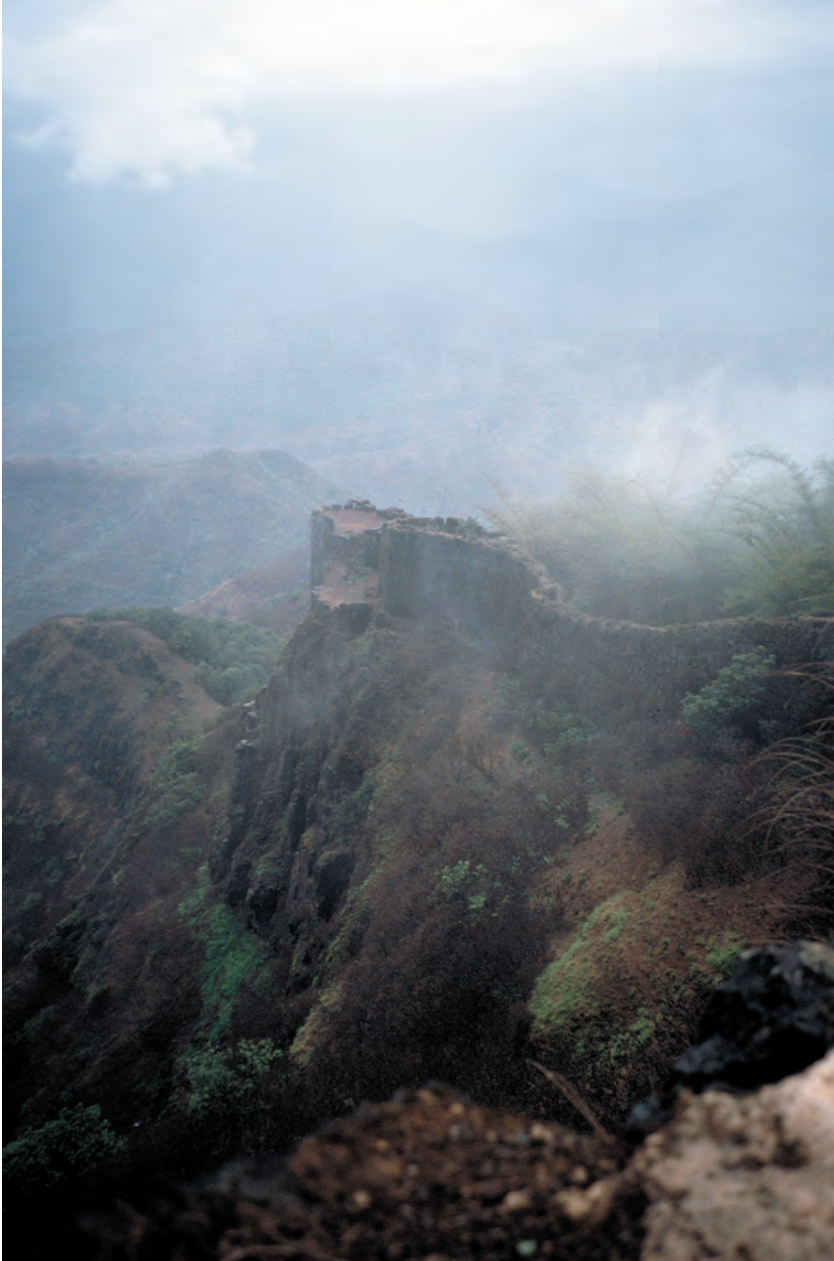
Plate 15. Pratapggarh: exterior walls and bastion, looking south.
