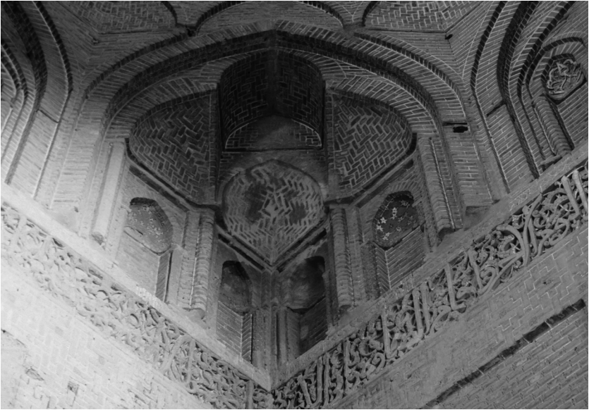
25.5 Zone of transition in the dome chamber, Great Mosque of Ardistan, Iran (early sixth/twelfth century). Photo: Marcus Milwright.
