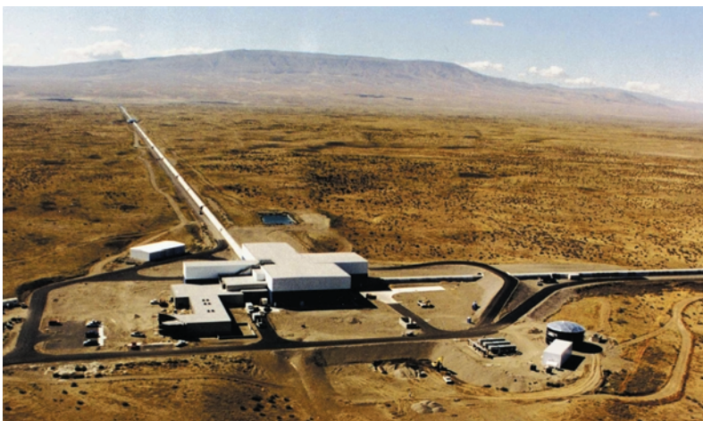
Fig 8.11. To detect gravity waves, physicists are hoping to measure very small changes in very large objects. This shows a view of one station of the Laser Interferometer Gravity Observatory (LIGO), in Hanford, WA. A passing gravity wave would cause a small shift in the interference patterns in the laser. [Photo courtesy of Caltech/LIGO]
