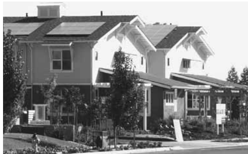
Fresno Cohousing has 1.5 Kw photovoltaic per house.
