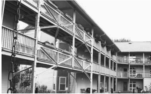
Bridge and balconies.
