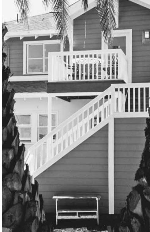
A new house built on top of an old, gutted and renovated one.
