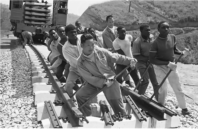
Figure 4. Building the Tazara Railway, 1967. From Beijing Review , http://www.bjreview.com.cn/special/2014-04/24/content_615209.htm .
