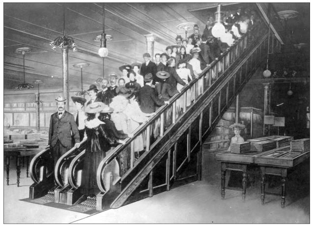
An Otis duplex cleat-type escalator, installed at the R. H. White Company store in Boston, Massachusetts, in 1903. (The Granger Collection, New York)
