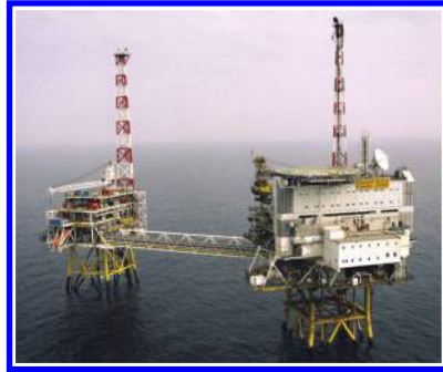
Figure 6.17: Draupner offshore oil field platform (from [6], photographed by Øyvind Hagen).
