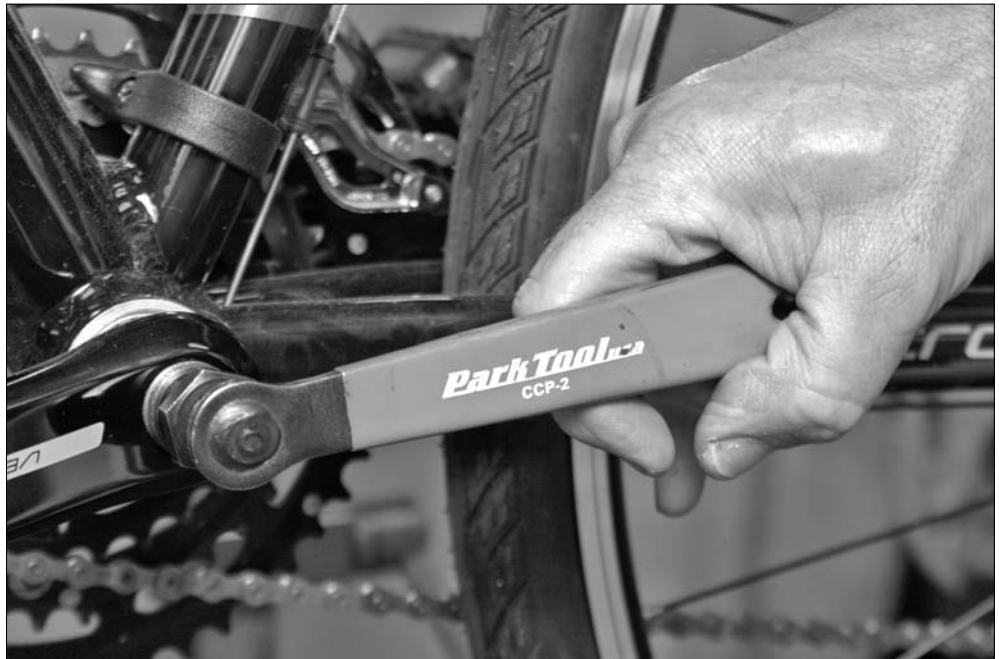
Figure 13-8: Using the crank-arm extractor.
