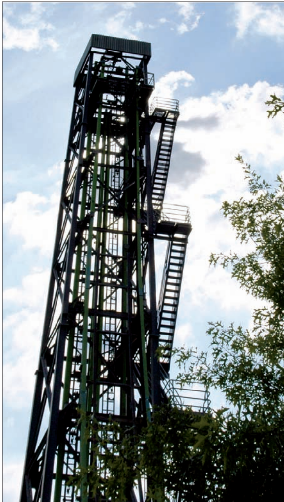
Figure 10-6: Tilt your camera back, and a tall structure appears to be falling away from you.
