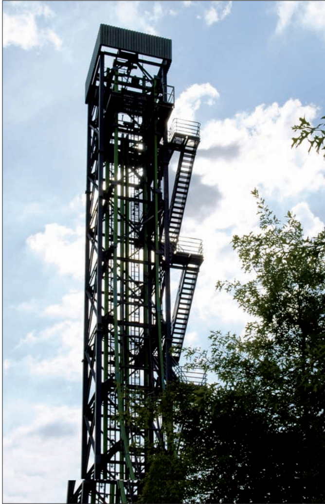
Figure 10-8: The corrected tower looks like this.
