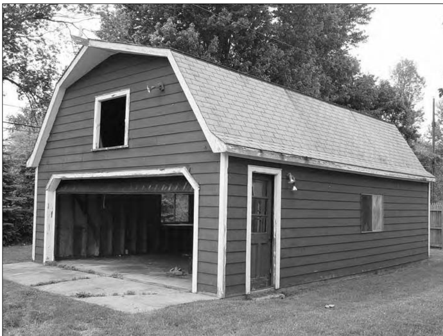
Figure 15-5: This garage looks disheveled.
