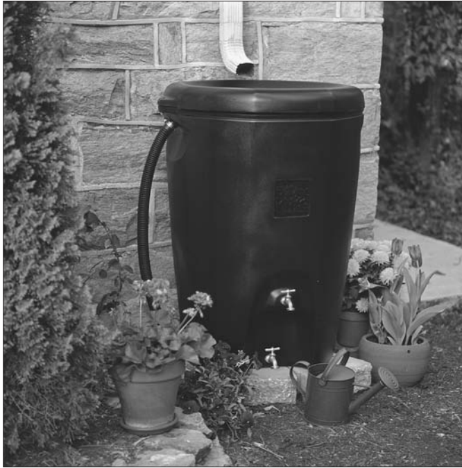
Figure 7-2: This rain barrel collects water from the building's roof.
