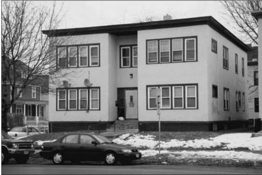
Figure 19-4: Before, the building looks dreary.
