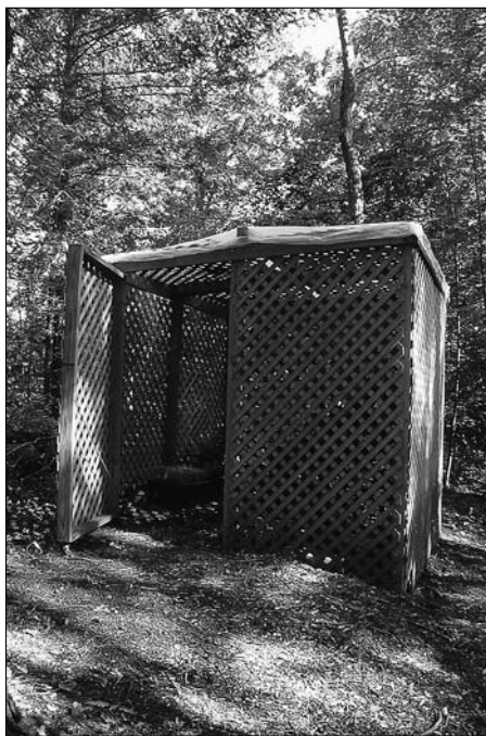
Figure 5-11: My shade house is an 8-foot (2.4-m) square simply constructed using wood lath and 4-x-4-inch (10-x-10-cm) pressure-treated wood posts.
