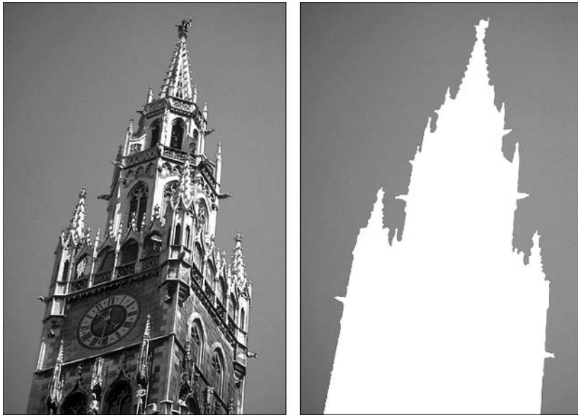
Figure 9-10: This building (left) is too darned ornate to select easily, but it's a snap to select the sky and then inverse the selection. Filling the selection with white (right) shows how accurate the selection is.
