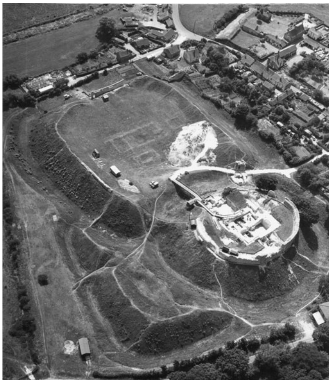
16. Castle Acre Castle, Norfolk, which belonged to the Warenne family. The original building of the 1070s was the stone house visible in the photograph, around which a much more substantial castle was constructed during Stephen's reign
