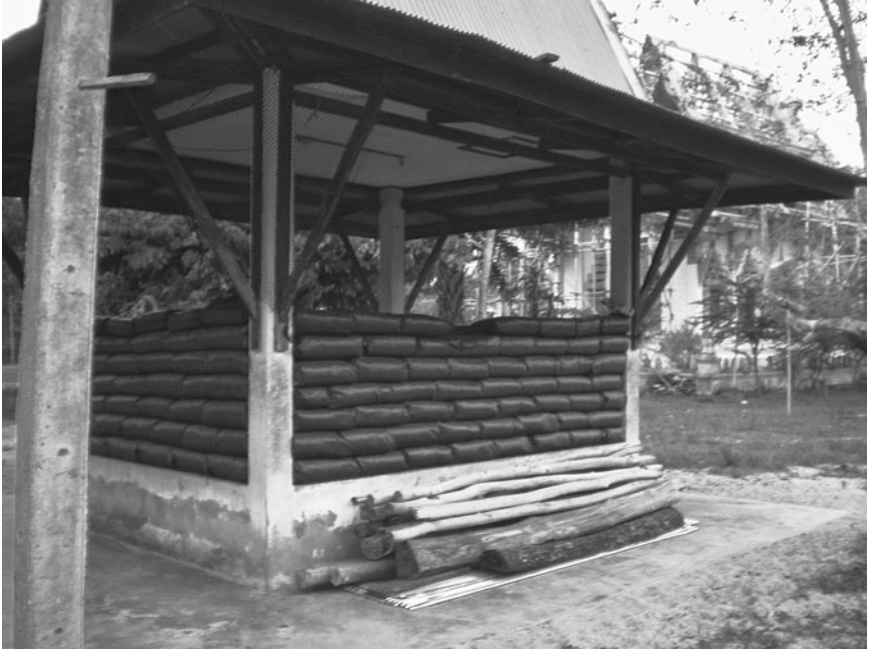
FIGURE 8.2 Thai pavilion converted into barracks within a Buddhist monastery. Photo taken by Michael Jerryson.
