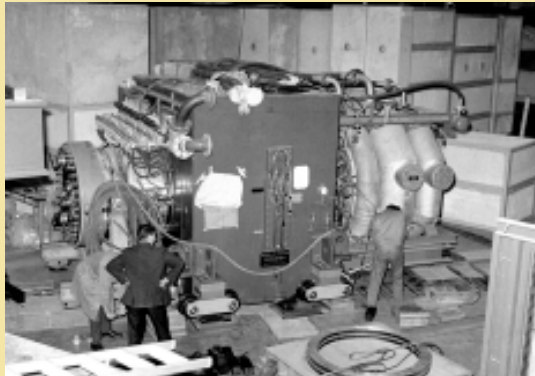
Installing the Heavy Liquid Bubble Chamber.
