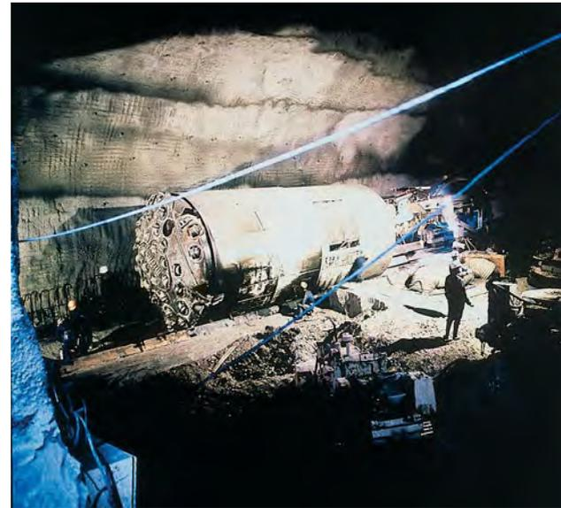
**Fig. 8.29** LEP’s 27 km long tunnel was excavated for the most part by three boring machines known as ‘moles’. These could bore rapidly, at about 25 m a day, through the sandstone of the plain around CERN, but blasting was necessary in some 3 km of harder rock at the foot of the Jura mountains. The ring was built with a tilt of 1.4% to keep as much as possible of the portion close to the Jura in the upper layers of softer rock.
