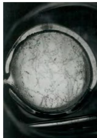
Fig. 6.24 The first tracks observed in liquid hydrogen, in John Wood's 3.5 cm bubble chamber in 1954.
