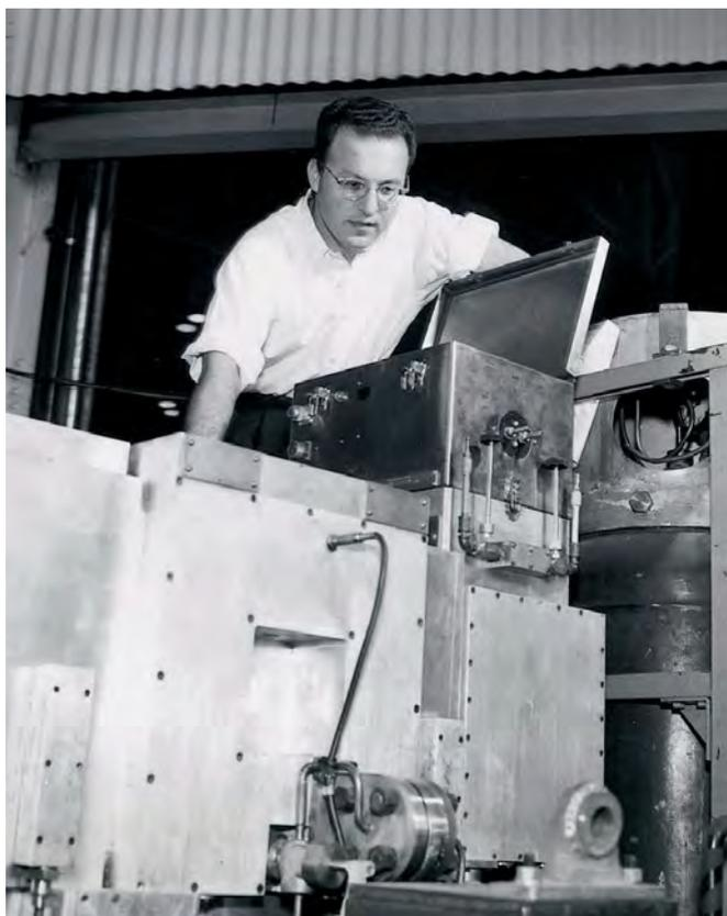
**Fig. 6.21** Donald Glaser (b. 1926) inspects a xenon bubble chamber at the Lawrence Berkeley Laboratory in the early 1960s. Xenon is useful because it forms a dense liquid in which gamma rays readily become 'visible' by converting to electron-positron pairs.
