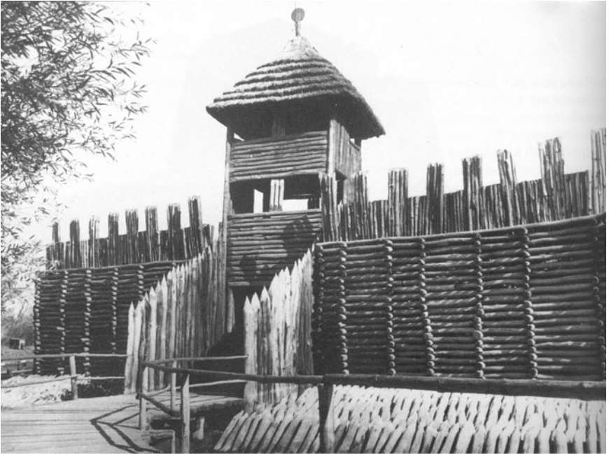
A reconstructed stockade around an early Iron Age settlement at Biskupin, Poland. Lausitz culture. As locally plentiful materials were utilized, wood, earth, clay-mud, and stone were variably used by pre-state societies in different environments around the world
