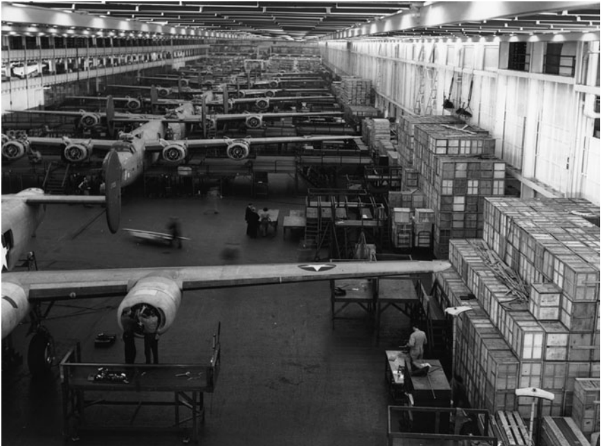
B-24 heavy bombers are mass produced in Ford's giant factory at Willow Run, Michigan
