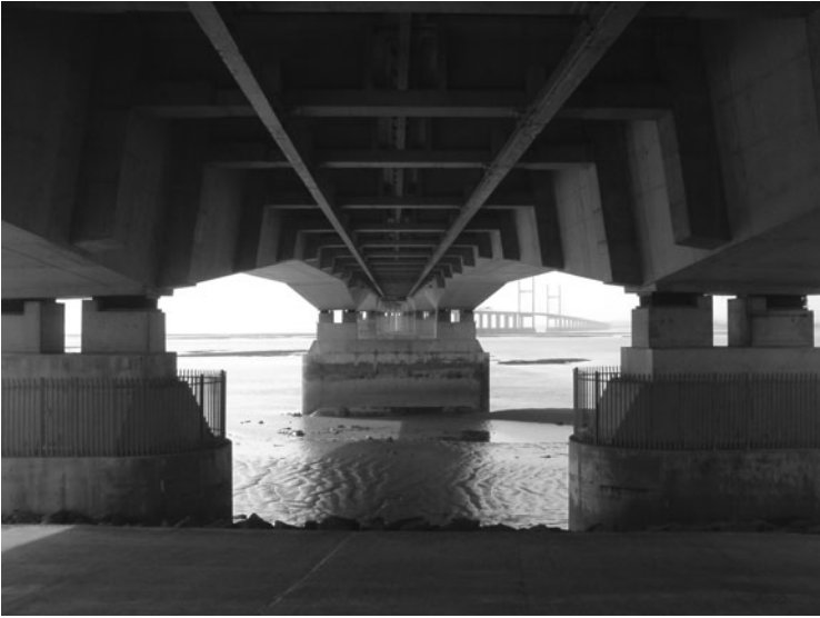
FIG 16. The underside of the Second Severn Crossing approach spans
