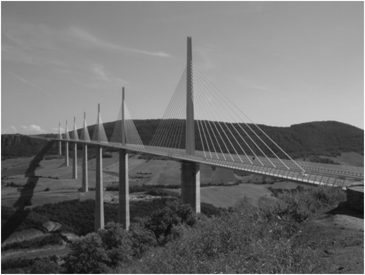
FIG 33. Millau Viaduct, France
