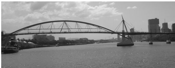
FIG 41. The Goodwill Bridge, Brisbane, Australia
