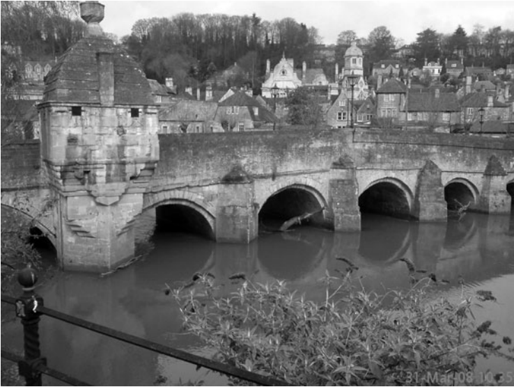
FIG 7. Masonry Arch Bridge at Bradford on Avon near Bath, UK
