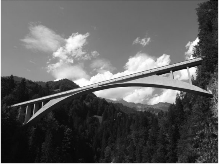
FIG 13. The Salginatobel Bridge, Switzerland
