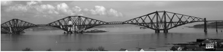
FIG 4. Forth Railway Bridge
