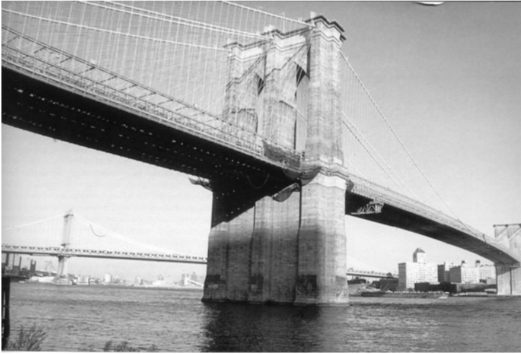
FIG 37. Brooklyn Bridge, New York
