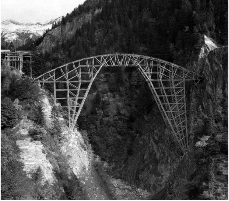
FIG 8. Centring for the Salginatobel Bridge, Switzerland
