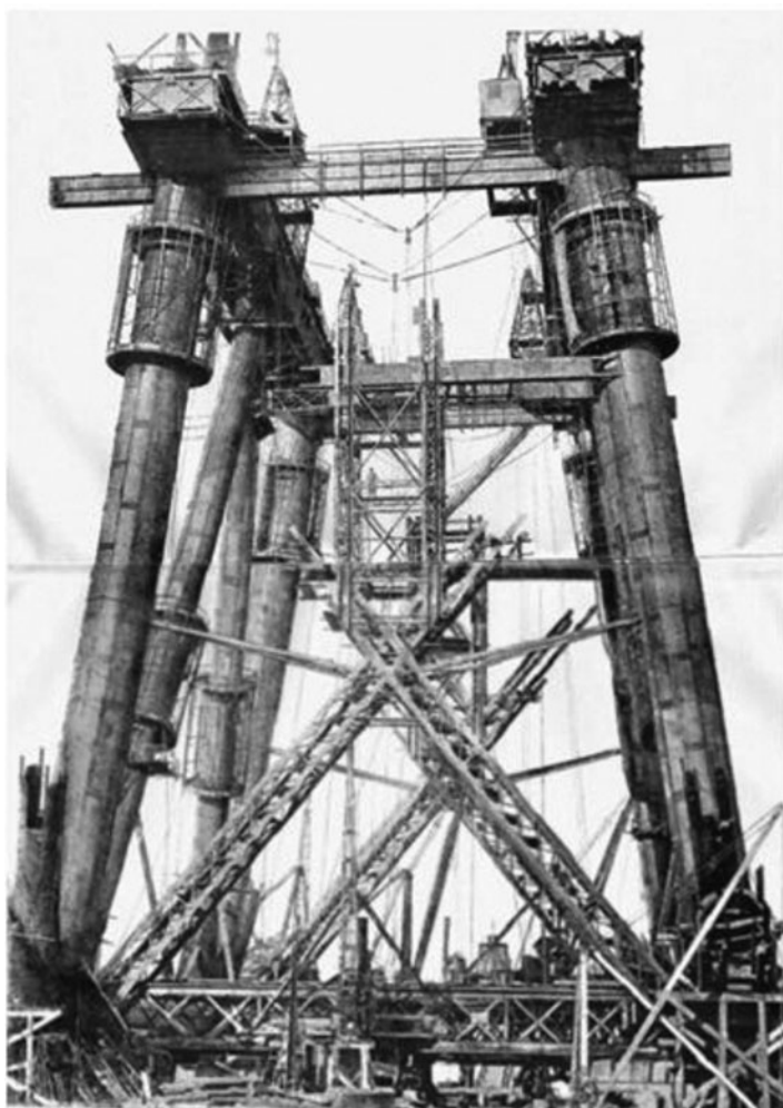
FIG 27. Erection of a leg of the Forth Railway Bridge
