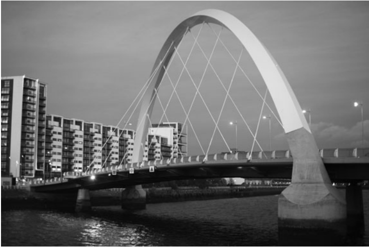
FIG 14. The Clyde Arc Finnieston Bridge, Glasgow
