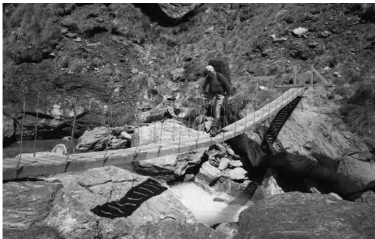
FIG 31. Snowy Creek Bridge, New Zealand
