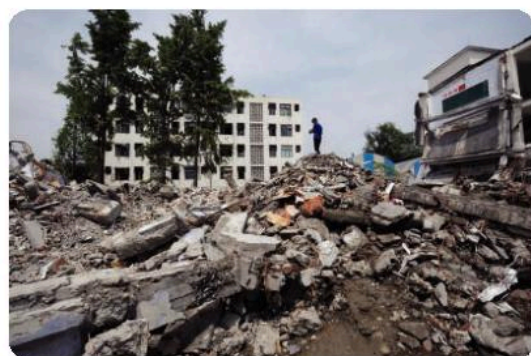
The remains of Juyuan Middle School in Dujiangyan, which collapsed in the earthquake. Around 900 students from this school were killed in the disaster.
