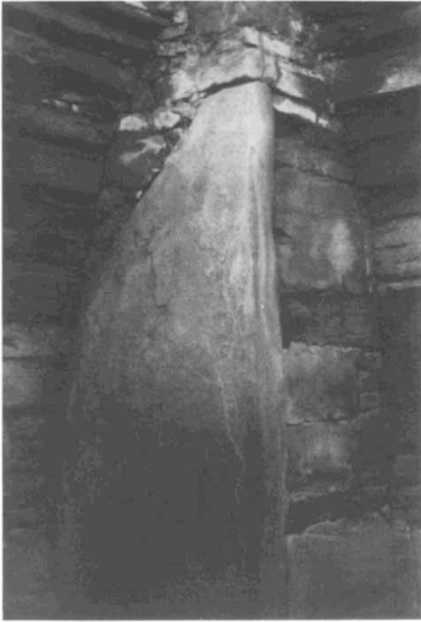
Plate 31 Maes Howe. One of the large, squinching buttresses in the central chamber
