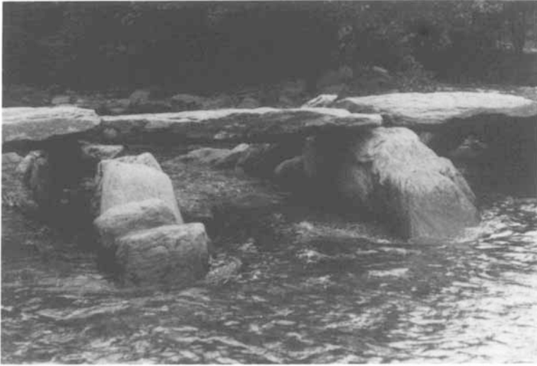
Plate 16 Tarr Steps. Some see this megalithic bridge as a medieval structure. It may well have been rebuilt several times following flood damage but it nevertheless lies on a neolithic route
