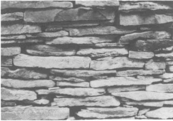
25 Drystone walling in the Unstan stalled cairn on Orkney. This is characteristic neolithic masonry, though here reconstructed, and often was used as an infill in megalithic architecture
