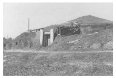
Figure 2.3 Ongoing reconstruction of Ocmulgee earthlodge. (Note exposed concrete and steel protective shell.)
