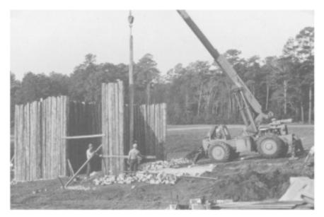
**Figure 2.13** Reconstruction using heavy equipment of wooden stockade wall at Andersonville
