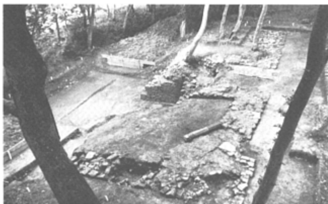
75 Foundations of the early-fourteenth-century stone-built gatehouse at Glottenham, in Sussex (Martin)
