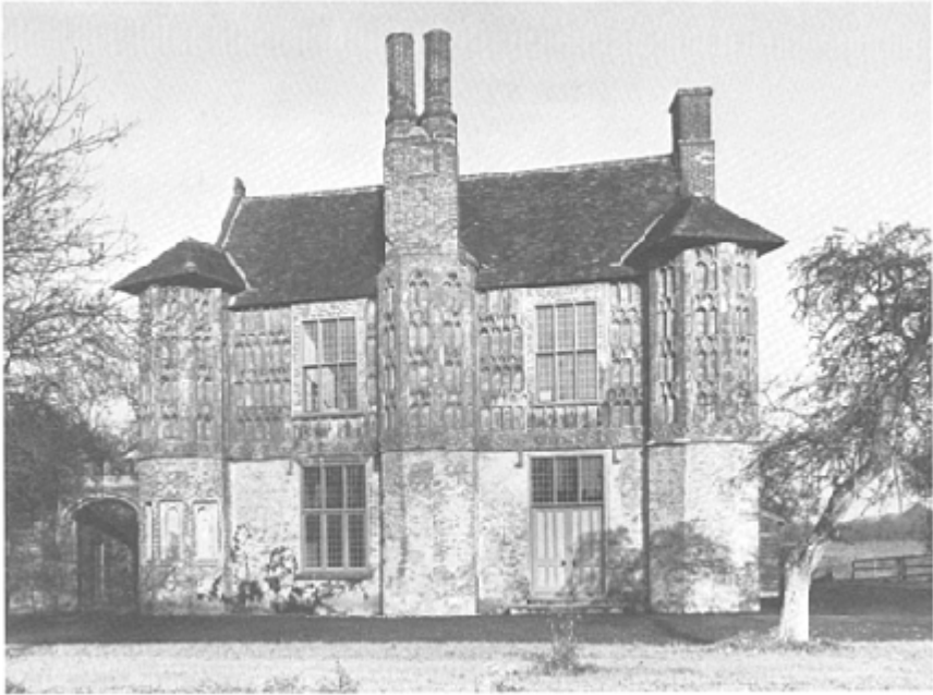
155 Sophisticated brickwork with terracotta panels at Great Cressingham Manor, Norfolk, a house of the 1540s (Hallam Ashley)
