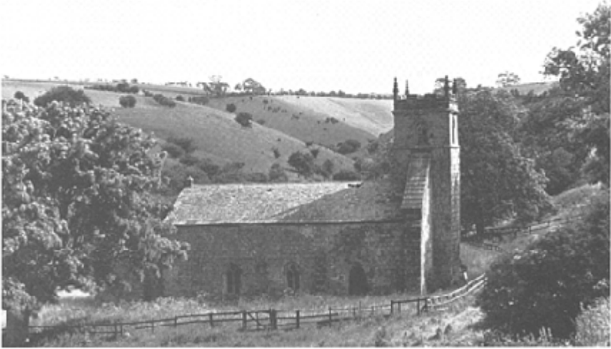
52 Wharram Percy Church, Yorkshire, showing the blocked arcading of the thirteenth-century north aisle, demolished in the later Middle Ages (R.C.H.M.)
