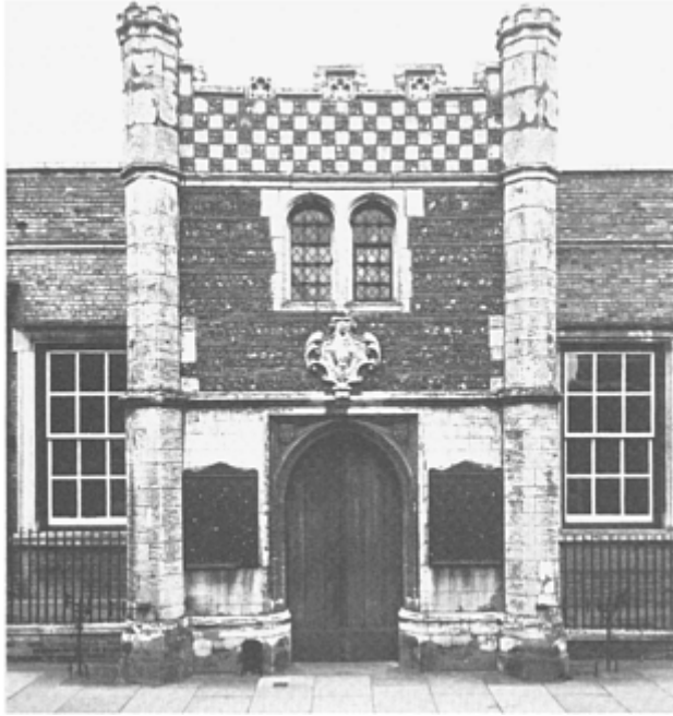
129 The porch, with first-floor 'Evidence House', of the guildhall at Bury St Edmunds; late-fifteenth-century (R.C.H.M.)
