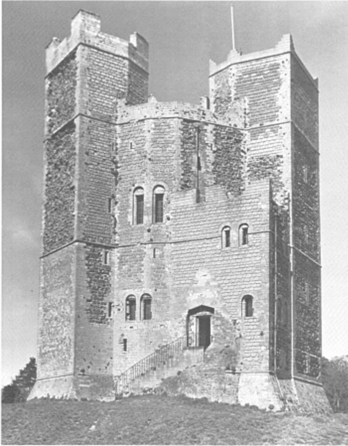
60 Henry II's polygonal keep at Orford Castle, Suffolk, built in the late 1160s as a counter to the Bigod fortress at Framlingham (Hallam Ashley)
