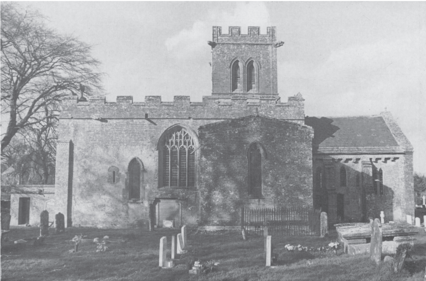
21 East Stoke church, Stoke sub Hamdon in Somerset. A good example of a medieval parish church with many building periods and styles represented. A highly-decorated elaborate Romanesque building of nave and chancel has had thirteenth-century tower and transept added. In the fifteenth century the nave was raised and battlements added. A new perpendicular church was not provided in the fifteenth century, as most local investment went to the now demolished St Nicholas chapel at West Stoke. (Photograph by Alan Wilson)
