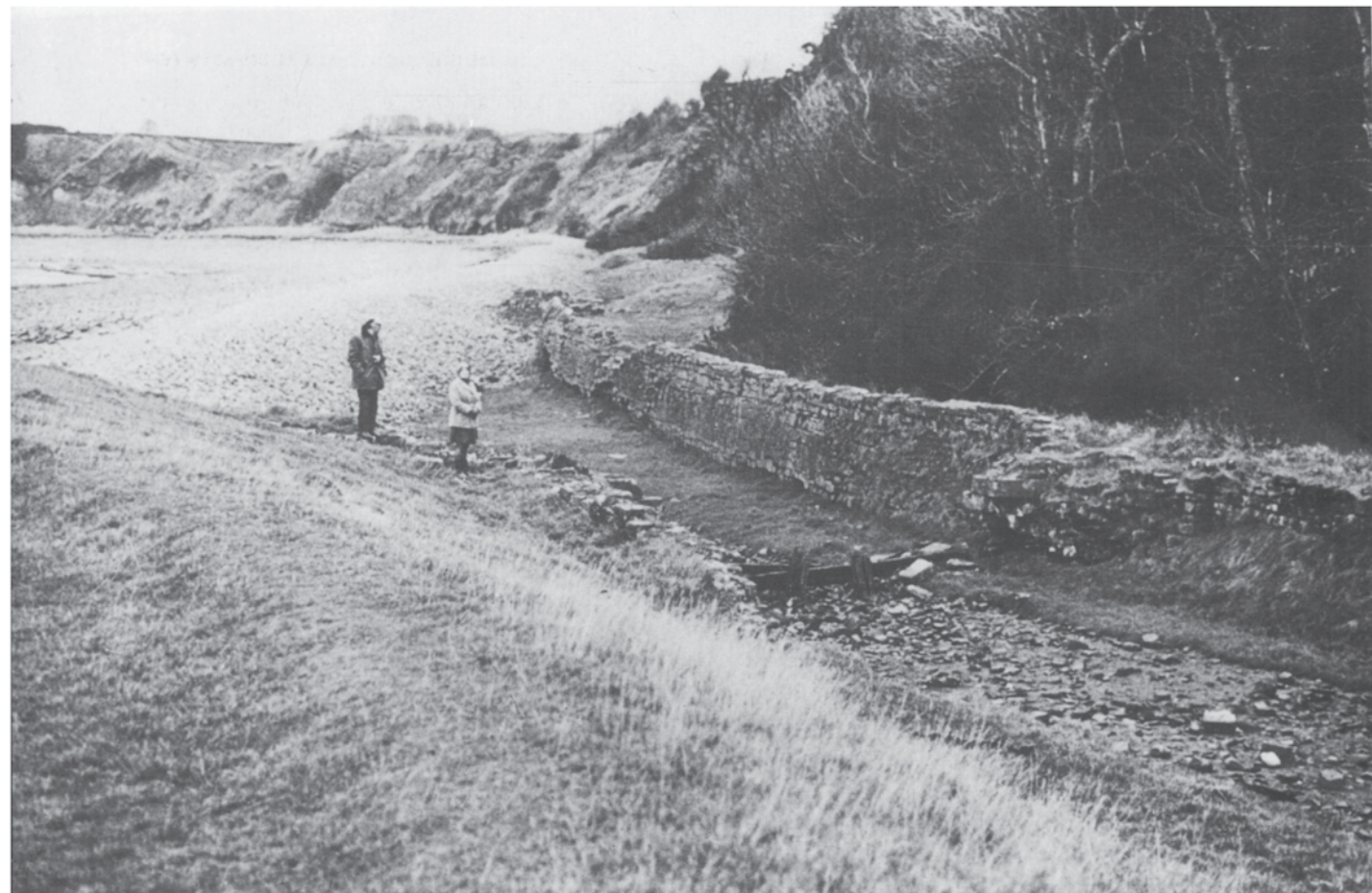
86 The abandoned harbour at Lilstock in Somerset. The entrance to the nineteenth-century harbour from the sea is now blocked by a bank of pebbles. Stone walls still line the dock and the remains of the harbour gates can be seen.
