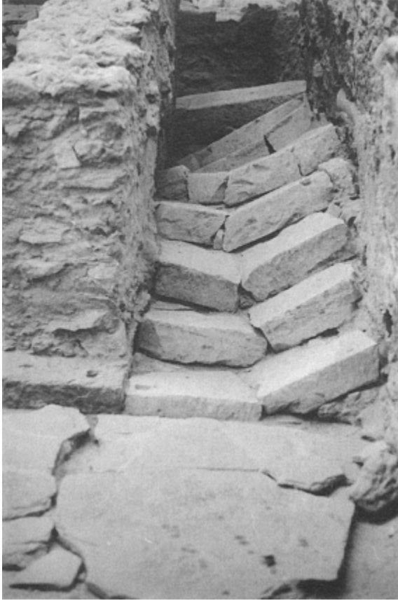
Plate 9.1 Staircase in Building 13 crushed during an earthquake: view from North Square
