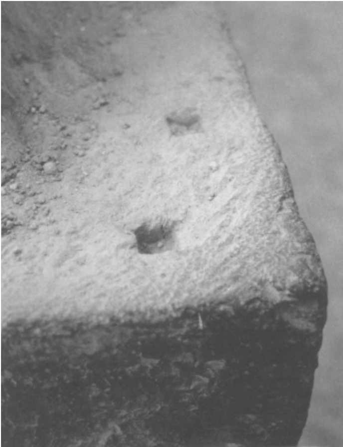
Plate 3.2 Minoan masonry techniques in use in Thera: cornerstones were fixed together with square bronze dowel pins, just as at Knossos
