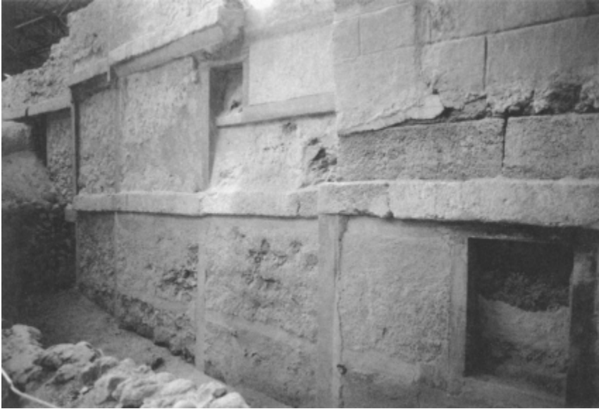
Plate 4.5 North wall of Building 17, still standing three storeys high, showing cornices and casts of timbers
