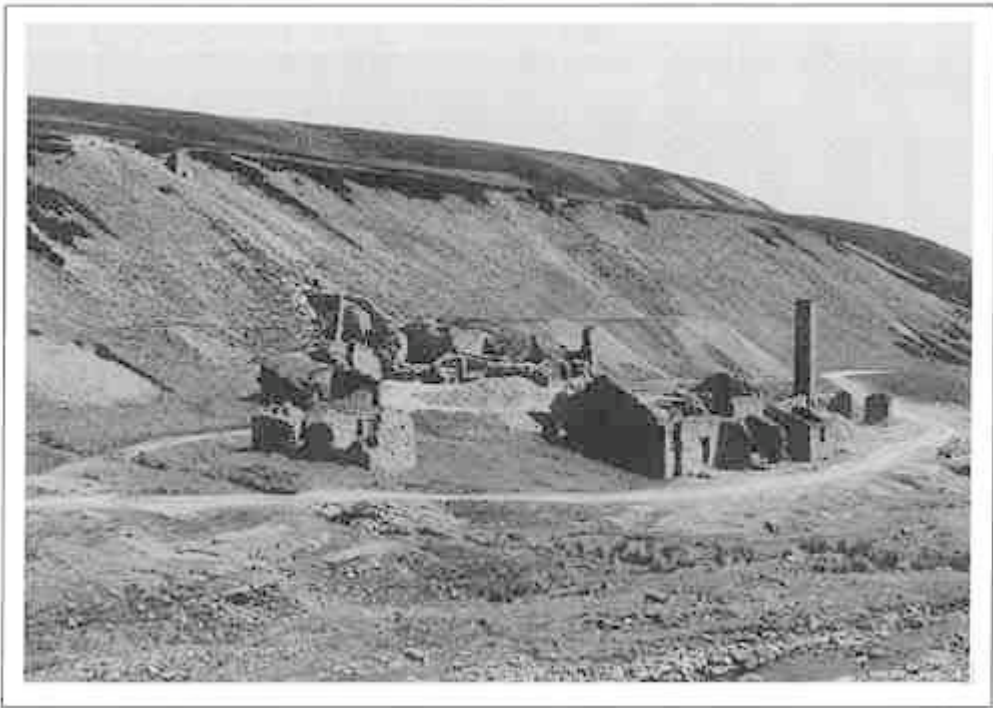
Plate 24 The derelict buildings of Old Gang smelt mill in Swaledale, North Yorkshire. Its situation in a valley bottom enabled the use of water power to operate bellows, whilst the valley side provided the route for the condensing flues linking the hearths to the remote chimney.
