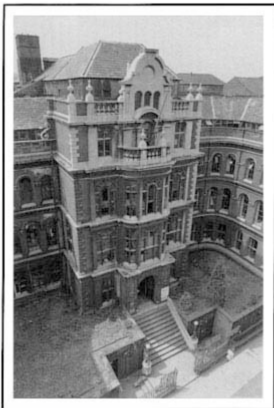
Plate 18 The warehouse built for Thomas Adams, a Nottingham lace manufacturer, one of several in the Lace Market. It was designed by a well-known local architect, T. C. Hine, with the intention of impressing visiting buyers, but also incorporated lace-finishing rooms in the attic storey, together with welfare facilities for the workforce.
