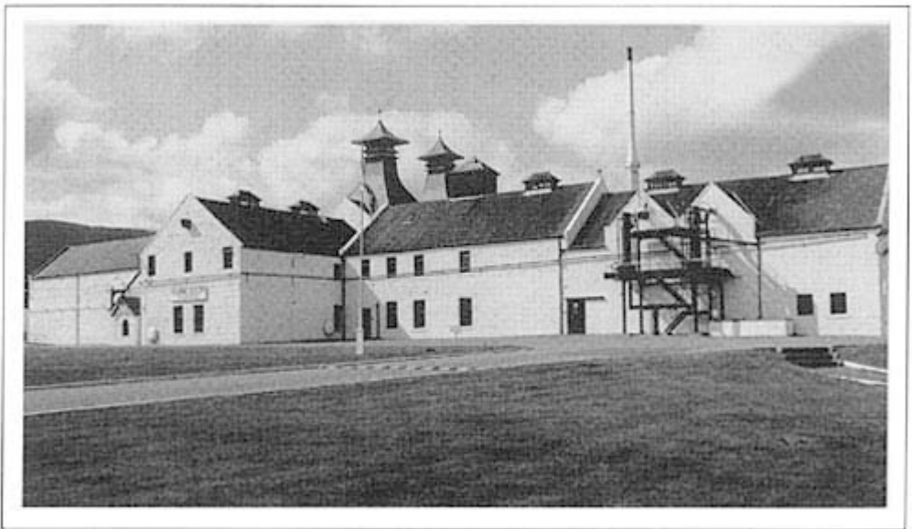
Plate 28 The whisky distillery at Dalwhinnie in Scotland, dating from the late nineteenth century. A range of low buildings, the roof-line of which is broken by the pagoda-like vents of the malt-kilns and the louvered vents over the still-rooms.
