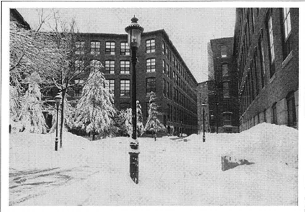
Plate 54 Some of the densely packed cotton mills in Lowell, Massachusetts, USA, converted to residential and office use and suitably landscaped.
