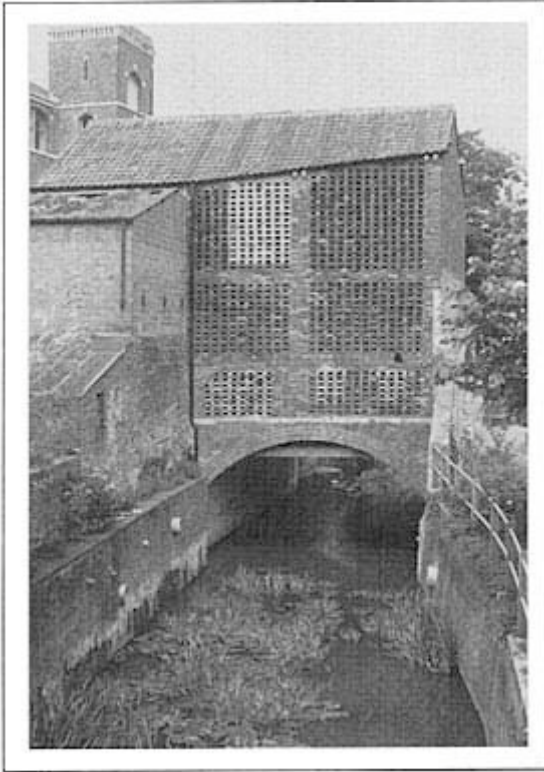
Plate 30 The ‘handle house’ at Studley Mill, Trowbridge in Wiltshire, a rare survival of a building characteristic of weaving communities. The perforations in the brickwork provided a draught of air for drying teasels after their use for raising the nap on damp woollen cloth.
