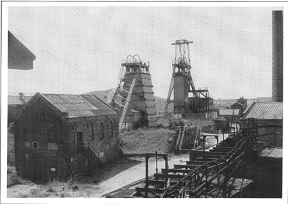
Plate 51 Three of the shaft head gears on the Chatterley Whitfield coal mine near Stoke-on-Trent in Staffordshire, only a fraction of a complex site whose conservation has posed major problems. The largest pit on the Staffordshire coalfield, it employed over 4,000 men at its peak. Unusually, it retains many of the ancillary structures such as a washery and heapsteads, which have been removed at other disused coal mines.
