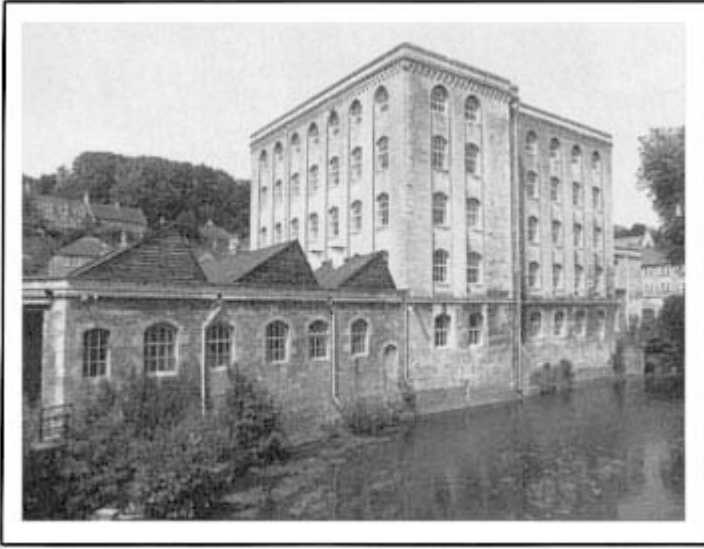
Plate 16 Abbey Mill, the last of the west of England woollen mills, was built in Bradford-on-Avon, Wiltshire, in 1874. It is an attractive stone building, with Gothic windows and an elaborate cornice: the original engine house can be seen on the right. The mill survived, like others in the town, through adaptive reuse for rubber manufacture and, more recently, for housing.
