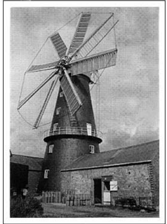
Plate 27 A rare survival of an eight-sailed tower mill at Heckington in Lincolnshire.
