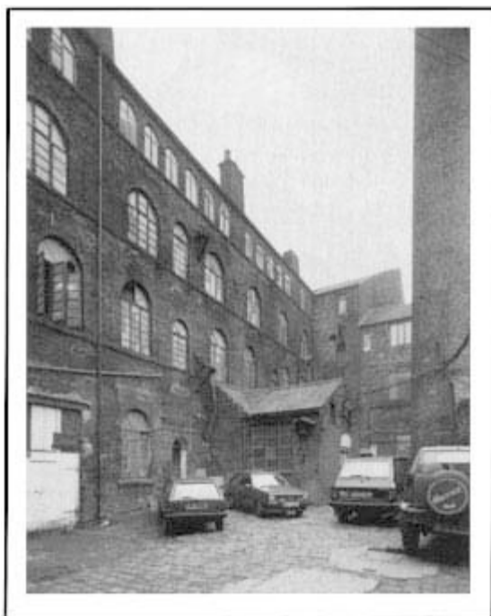
Plate 15 The multi-storey workshop complex known as Butcher's Wheel in Arundel Street, Sheffield, South Yorkshire. Three boilers in the courtyard supplied steam to three engines which provided power for the grinding wheels and other machinery. (See Figure 50.)
