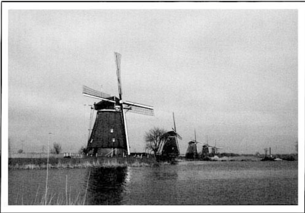
Plate 4 In no other place in the world can a landscape of windmills be more appreciated than at Kinderdijk, north of Dordrecht in the Netherlands. Two ranges of tower drainage mills, eighteen in all, lift water by means of scoop wheels from the Alblasserwaard polders into channels which flow into the River Lek.
