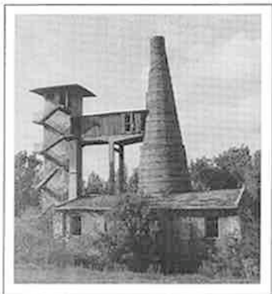
Plate 25 A sophisticated conical lime-kiln at Sulejow in Poland, which was at work until the 1980s. The kiln was charged by means of a lift in the adjacent concrete tower.
