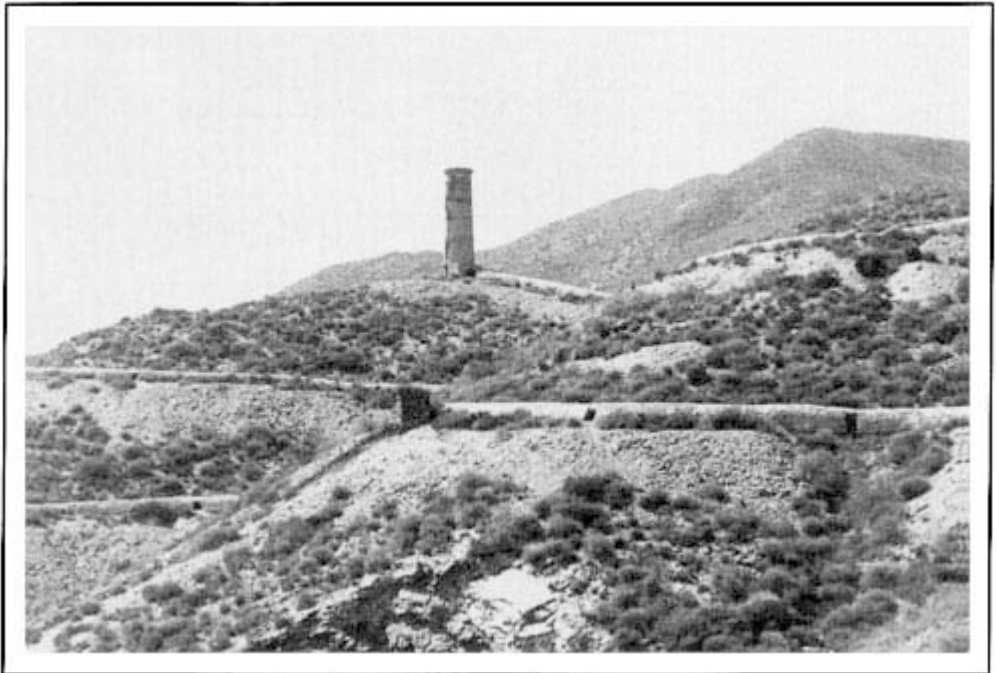
Plate 7 The extensive lead-condensing flues snaking across the barren landscape of the Sierra de Almagrera in southern Spain.
