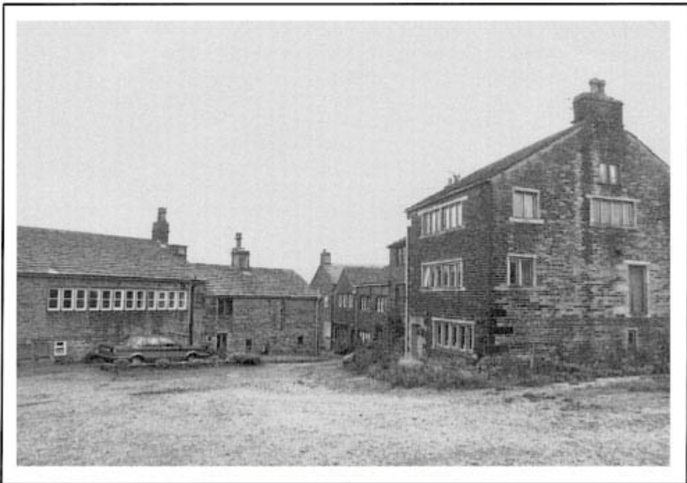
Plate 14 A typical weaving fold at New Tame, Delph, in the parish of Saddleworth in Greater Manchester. Around the nucleus of a seventeenth-century farmhouse, itself adapted for weaving by the insertion of long mullioned windows, a series of cottages with loomshops was added in the late eighteenth century. The three-storey building in the right foreground had a top-floor loomshop, while the 'taking-in' door on the middle floor enabled yarn to be received for weaving without intrusion into the ground-floor living quarters.
