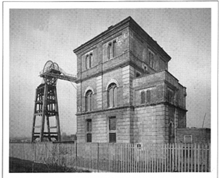
Plate 47 The now isolated vertical steam winding engine house and headstocks of the former Bestwood Colliery in Nottinghamshire. RCHME © Crown Copyright.
