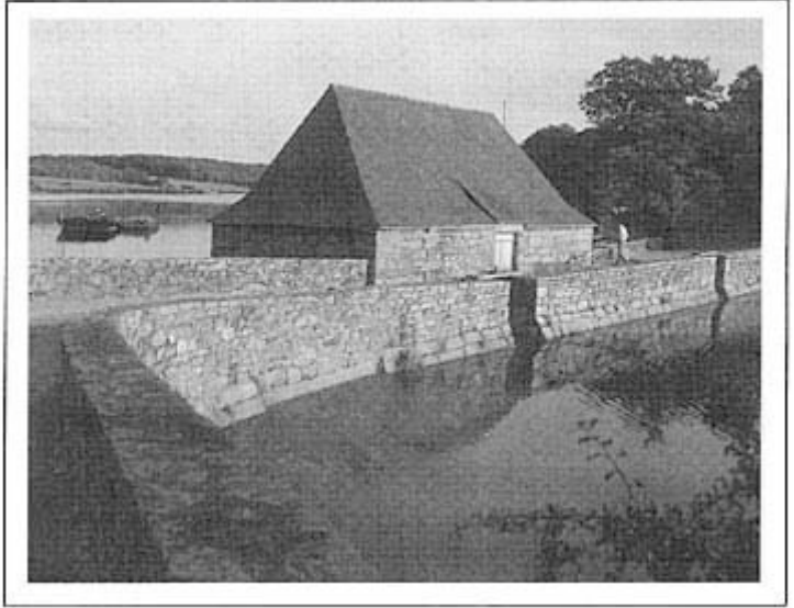
Plate 26 A squat stone-built tide-mill on the Gulf of Morbihan in Brittany, France. The mill is built into the causeway which also serves as the water storage dam. The two sluices, one for filling the pond and the other providing the feed to the waterwheel, can be seen.
