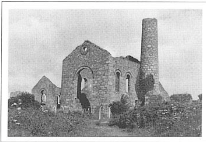
Plate 39 The pumping engine house at Marriott's shaft, Basset Mines, Cornwall, with the fenced shaft in the foreground. There is clearly no conventional bob-wall to support a rocking beam. The foundations within the engine house indicated the use of an inverted beam engine which was supported by loadings at first-floor level. Subsequent research showed that the house had been intended for two Davey compound engines, only one of which was installed in 1898.
