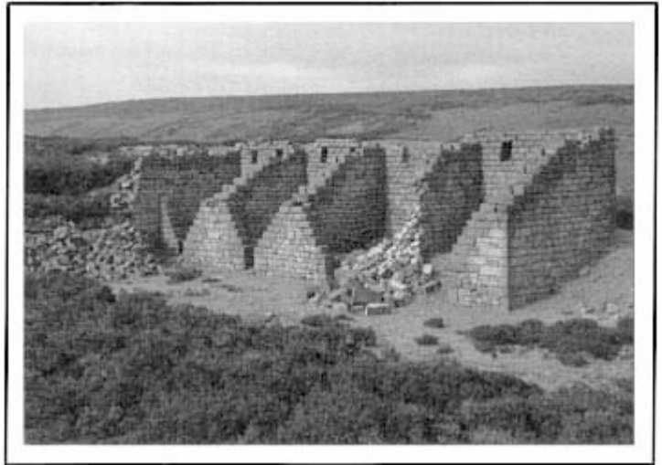
Plate 13 The row of ore storage bins at High Stoney Grooves lead mine in North Yorkshire. These were also known as bouse teams, since they served to keep separate the bouse, or ore, raised by each team of miners.
