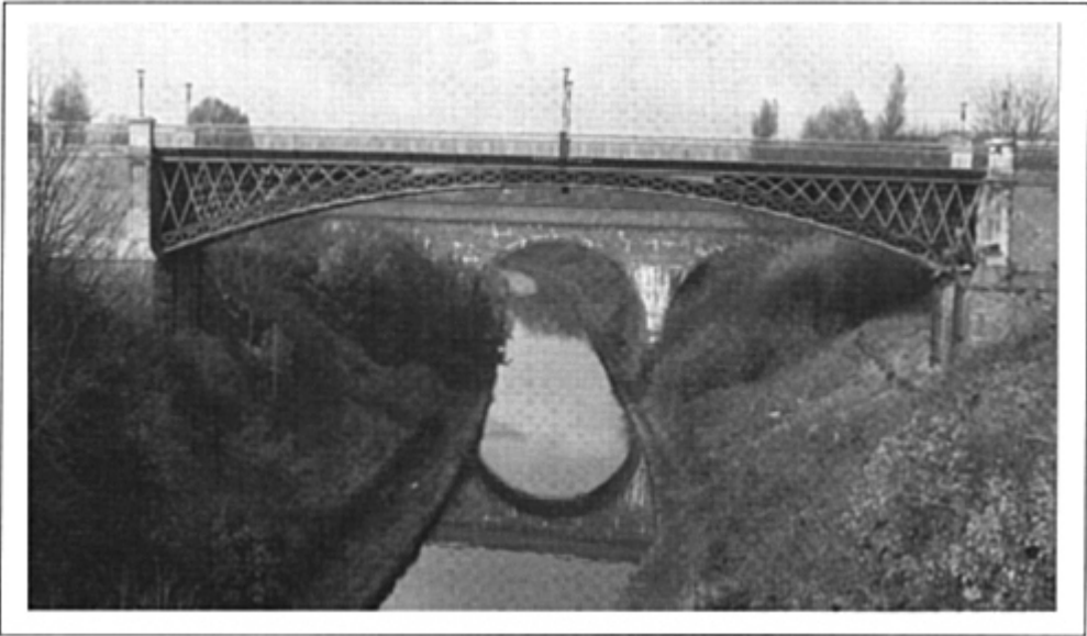
Plate 59 Telford's improvements to the line of the Birmingham Canal in the Galton Valley near Smethwick, West Midlands, resulted in a deep cutting which presented problems in bridging it. His solution was this magnificent cast-iron bridge of 1829.
