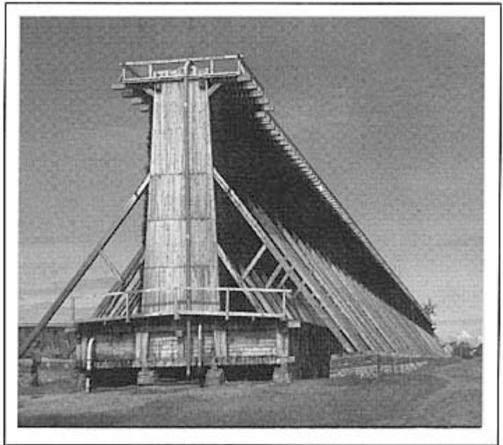
Plate 29 A rare survival, the massive wooden structure of the salt gradation tower at Ciechocinek in Poland.
