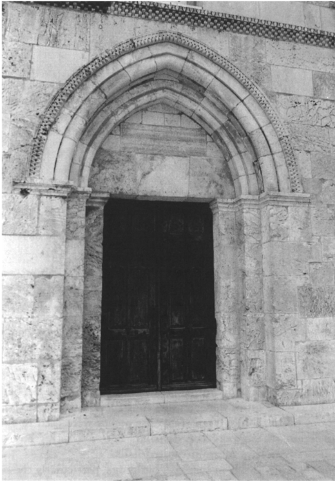
Plate 8.4 Moulded arch on the door of St Anne's Church, Jerusalem (photograph by Yael Sternheim)
