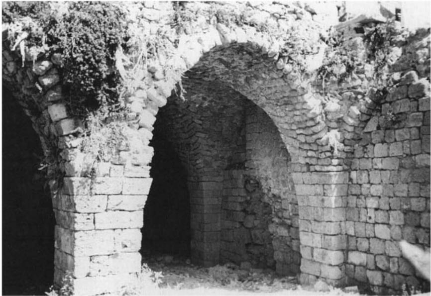
Plate 2.9 Akko: ground-floor vaults of a communal house in the Pisan Quarter (photograph by the author)
