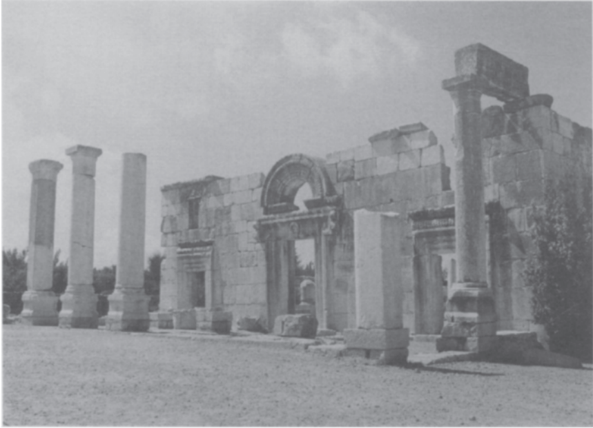
Figure 4.3 The facade of the Galilean synagogue of Bar'am
