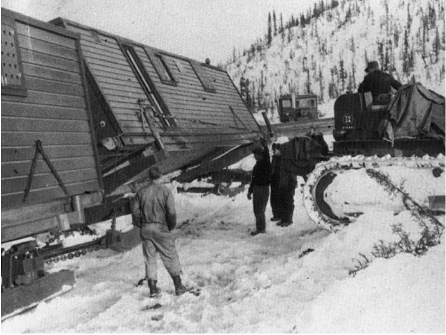
Figure 19.2 Modular buildings under construction for DEW Line station
