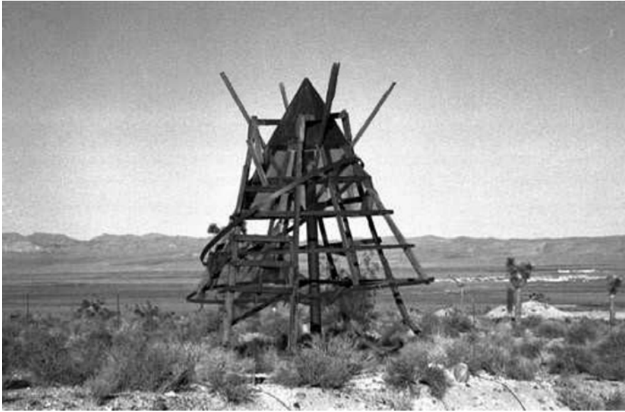
Figure 7.3 Electromagnetic pulse tower used in atmospheric nuclear tests
