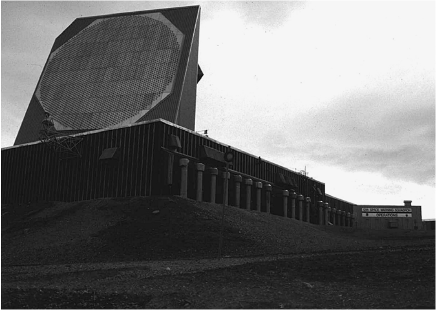
Figure 19.3 Upgraded radar facility at Thule Air Base, Greenland
