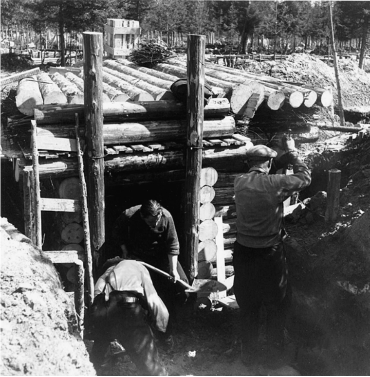
Figure 5.5 Civil workers building a typical Finnish wooden dugout
