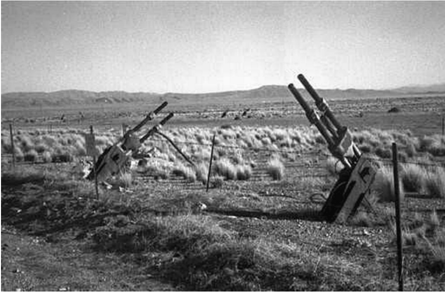
Figure 7.1 Stanchions that supported a tower for an atmospheric nuclear test
