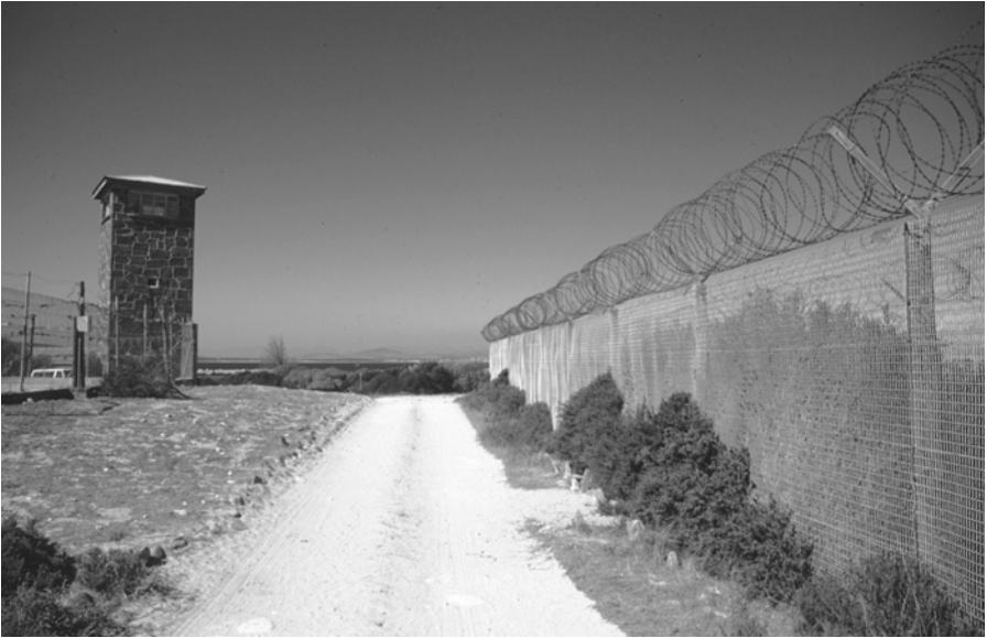
Figure 23.2 Although the prison buildings are the focus of attention on the island, it is important to remember that there is a ‘prison landscape’ which is as significant but which poses many management challenges
