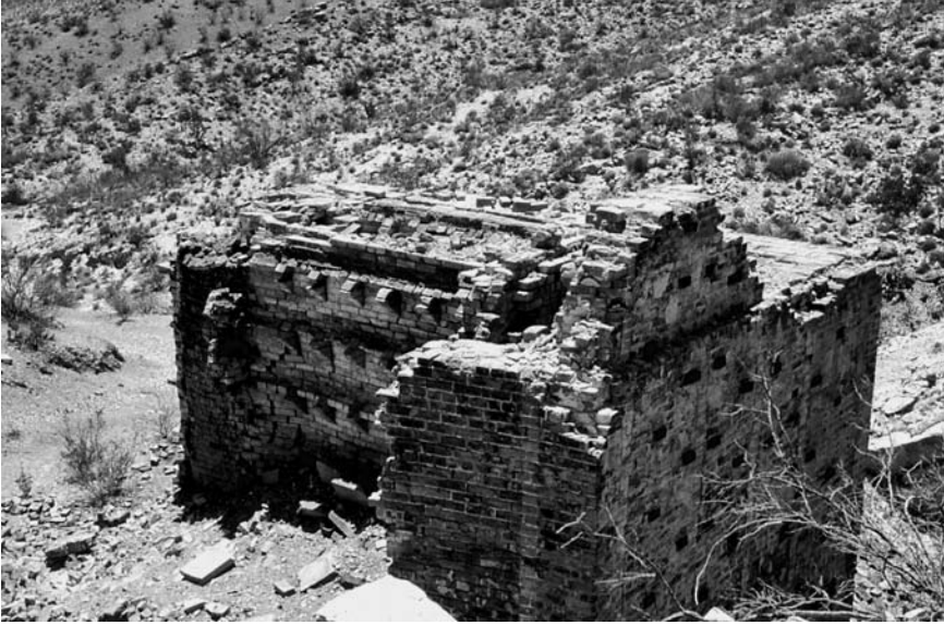
Figure 5.4 A Scott furnace, used to extract mercury in the early twentieth century, at the Mariscal Mine, Big Bend National Park, Texas
