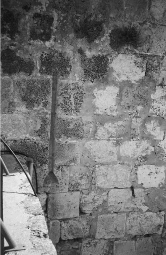
Figure 65 Stirrup-shaped arrow-slit at Doc (photograph by the author).
