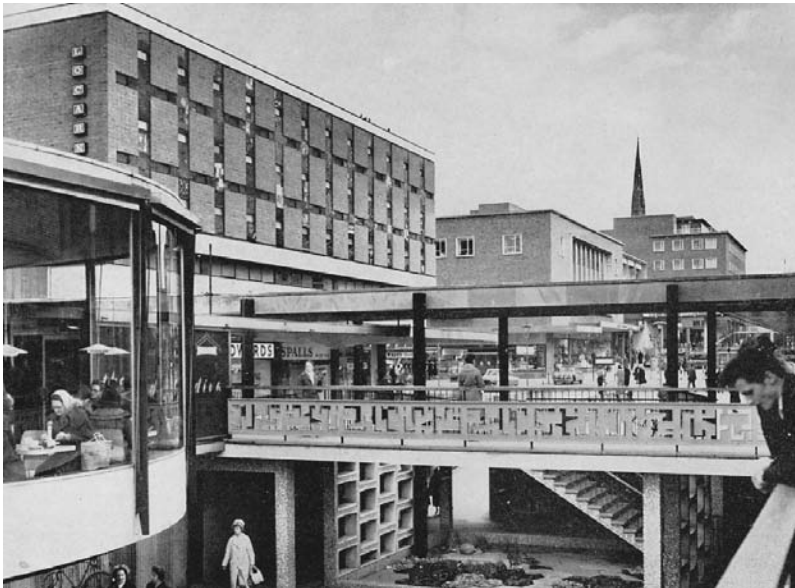
Plate 3.5 Post-war planning – exemplified here by Coventry city centre, UK – created multilevel precincts in which a maze of underpasses, overpasses, ramps and stairs created particular problems for parents and elderly people (see Hubbard and Lilley 2004)
