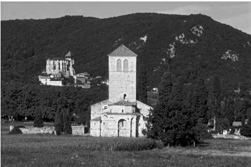
Figure 5.5 Saint-Just from the east with the upper town
