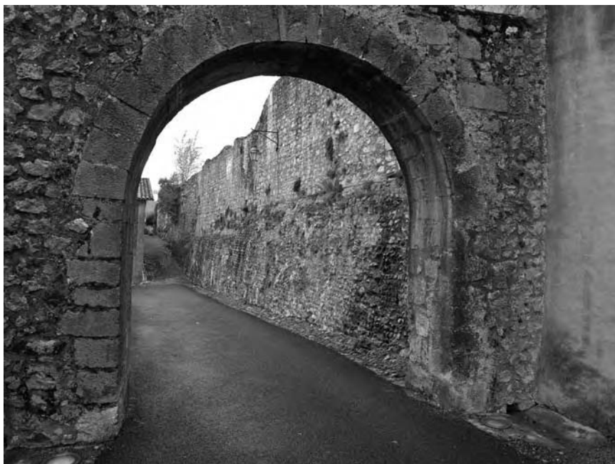
Figure 3.5 Hilltop, the terrace wall (lower part Roman, upper part medieval)
