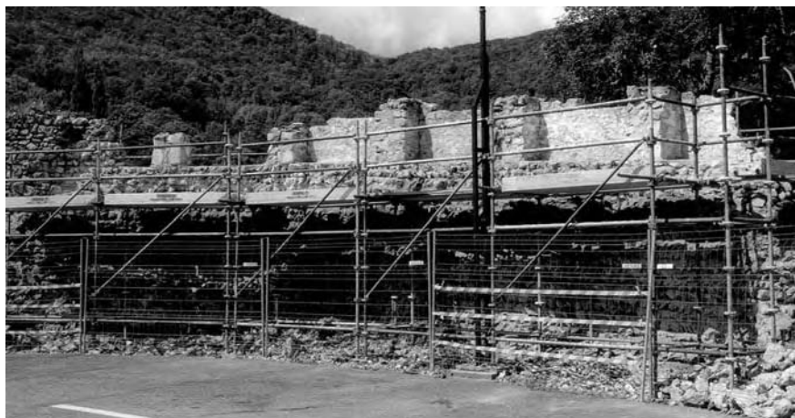
Figure 5.2 The wall-top with the walkway, parapet and traverses
