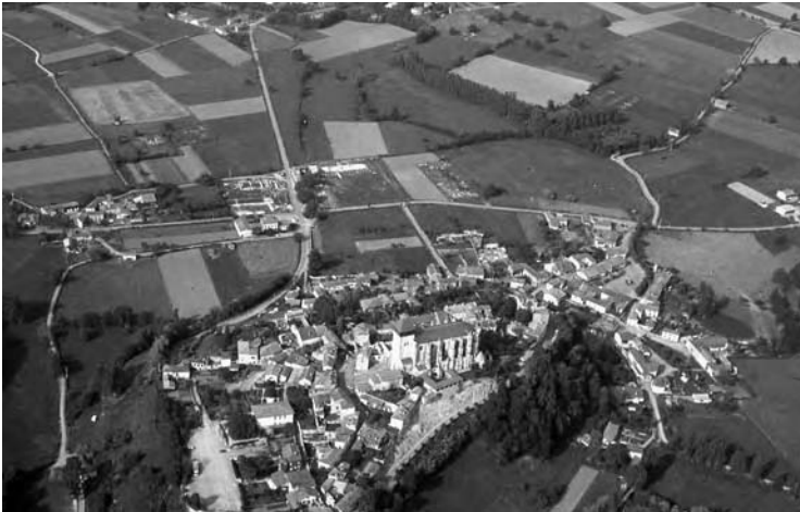
Figure 5.1 The upper town from the air: in the centre of the photograph the monuments of the centre of the lower town (© C2RA, Musée archéologique Saint-Bertrand-de-Comminges. Photo: Catherine Petit)
