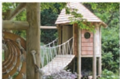
Install a playhouse and walkway.
