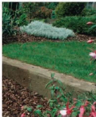
Use railroad ties to level shallow slopes.
