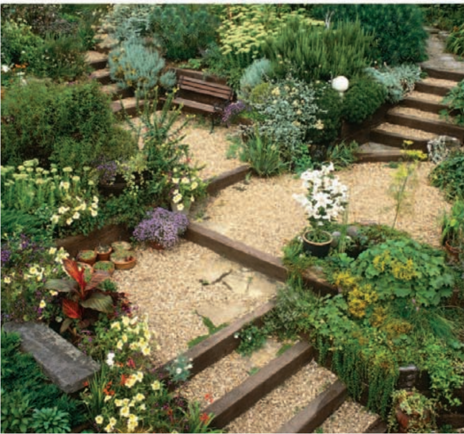
Use railroad ties to level shallow slopes.
