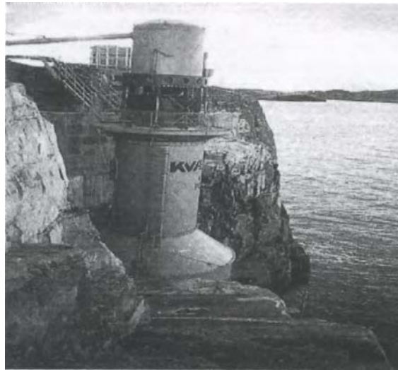
Top: Fig. 9.1 Kvaerner OWC (sectional drawing); Bottom: Fig. 9.2 Kvaerner OWC (Toftestallen demonstration plant)
