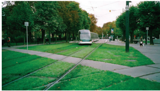
Fig. 18.6. Improving public transport with a modern light railway system to reduce our car dependency. Pedestrian friendly landscaping is possible with integrated light railway tracks.
