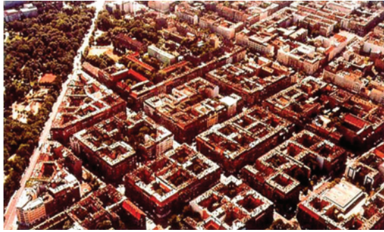
Fig. 18.1. The block model of the European city: five-storey blocks as found in Paris, Berlin, Barcelona, and in other cities, have proved a solid model for energy efficiency and dense living. These cities possess already the urban characteristics of a compact city model. The strategy of saving from passive-building technology is well accepted: a compact built form with a high level of thermal insulation reduces energy losses through transmission.
