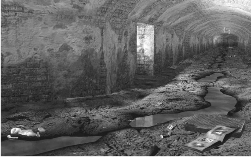
Figure 1. Objects in DarkCon culvert that show evidence of civilian usage.
