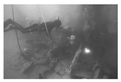
**Figure 9.18** Using a thermal lance (oxy-cutting equipment) to separate the engine from the boiler on the steamship *Xantho*. (Courtesy of Jon Carpenter, Department of Materials Conservation, Western Australian Maritime Museum.)
