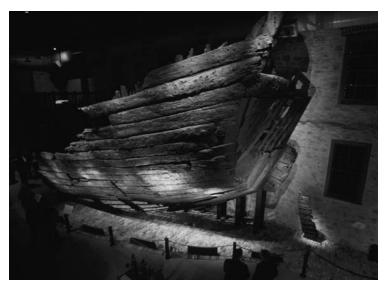
**Figure 13.4** The reconstructed timbers of the *Batavia*, Western Australian Maritime Museum, Fremantle. Only a small portion of the hull structure survived and this was dismantled *in situ*, raised, recorded, conserved, and then rebuilt.
