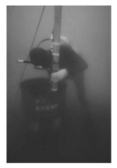
Figure 9.7 Caisson excavation using a 200-L fuel drum open at both ends, Takashima, Japan.
