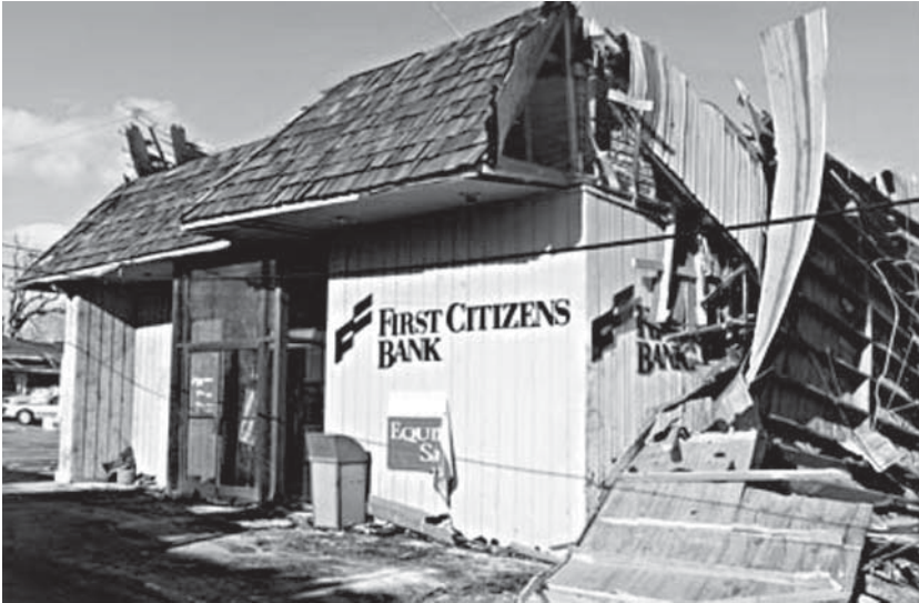
This North Carolina bank suffered major damage in a 1998 tornado. Researchers are increasingly turning their attention to the ways in which disasters affect private-sector organizations and to private-sector disaster preparedness.
