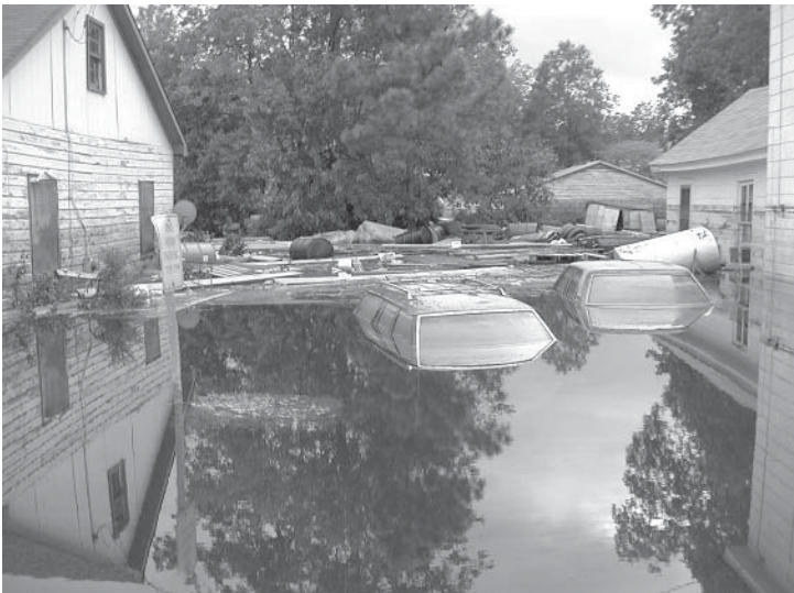
Hurricane Floyd left the downtown section of Franklin, Virginia, under six feet of water in September 1999. The water finally receded, but remaining hazards included propane tanks, gas tanks, chemical barrels, and pesticides.
